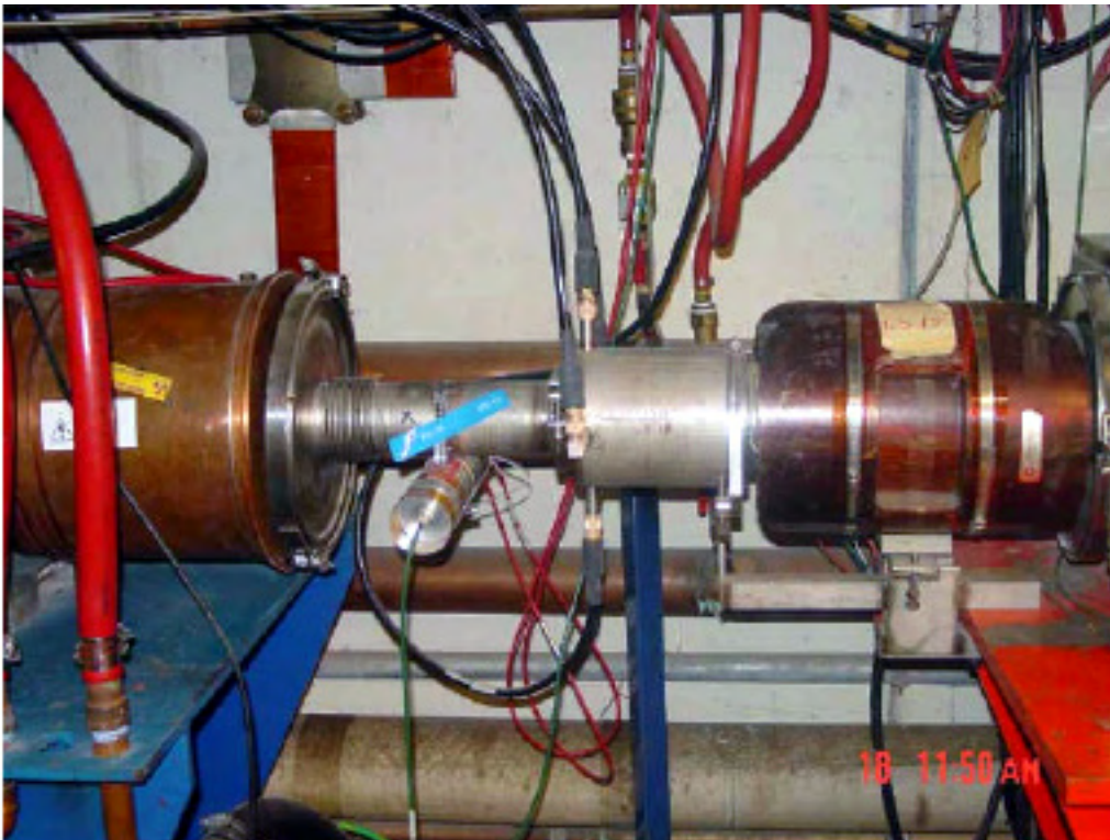
Exhibit 4-19: Booster Water Tube Replacement.
