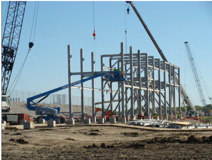
Revamp area (North-South piperack tank S-103) (24-Oct-2013)
