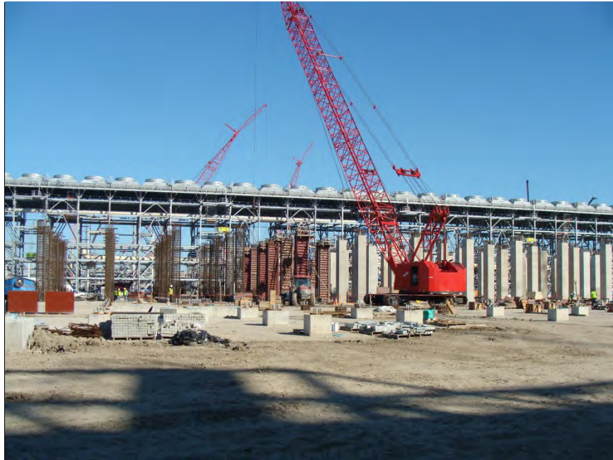
Train 2 (compressor columns) (24-Oct-2013)
