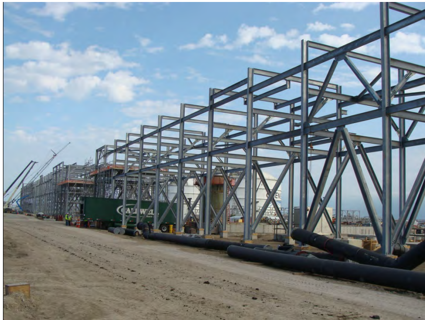
OSBL (pipe rack utilities) (18-Nov-2013)
