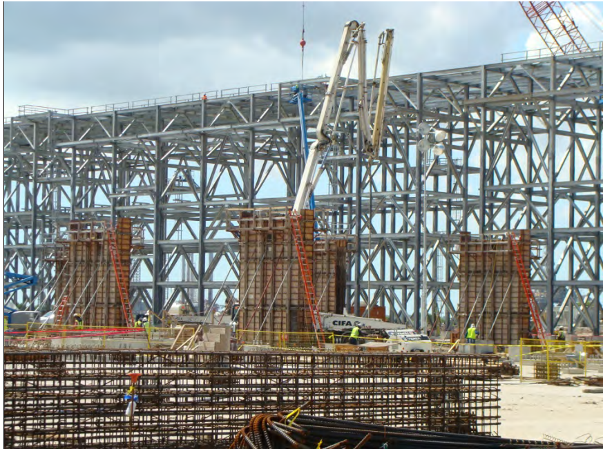
Train 2 132J01 (propane refrigeration) (24-Sep-2013)
