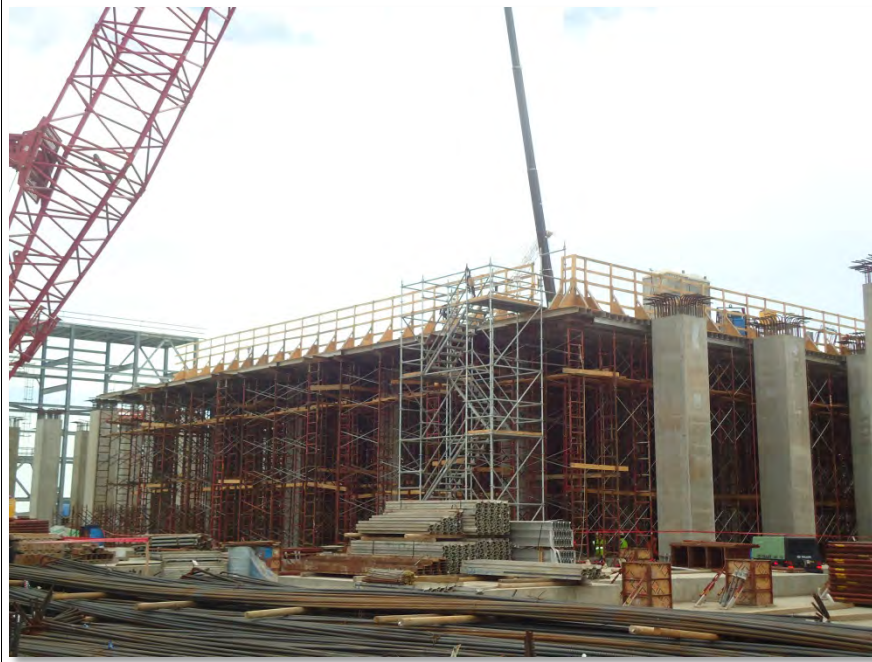
Train 1 131A01 (compressor area ethylene shoring) (12-Sep-2013)
