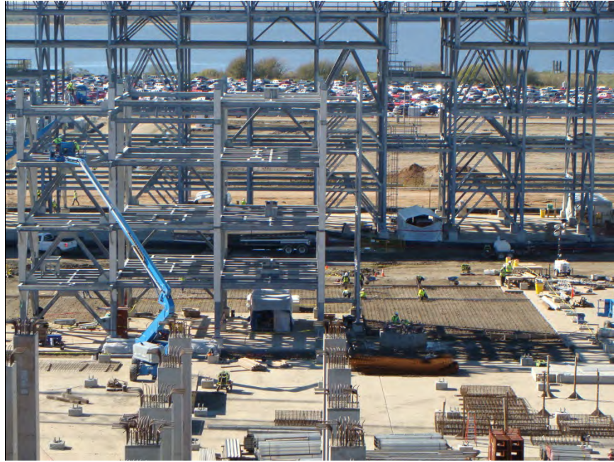
Train 2 (HRU unit paving)
