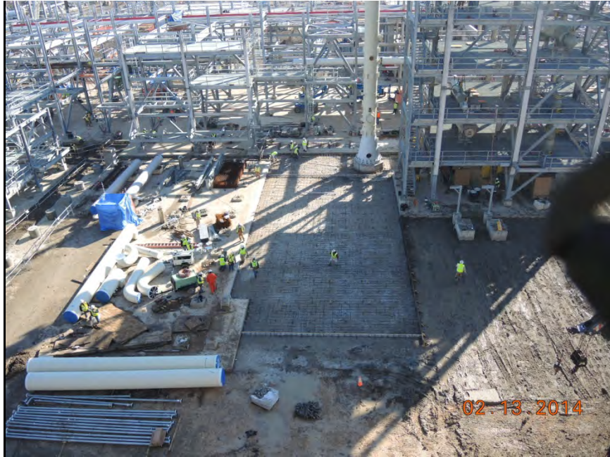
Train 2 131M01 (heavies removal unit paving) (13-Feb-2014)
