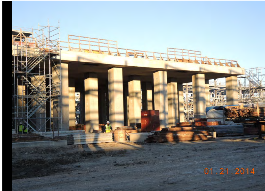
Train 1 131A01 (compressor tabletop shoring removal complete) (21-Jan-2014)
