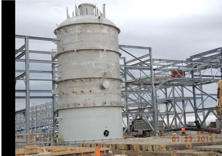
OSBL 135E01 (BOG compressor nitrogen drum) (23-Jan-2014)
