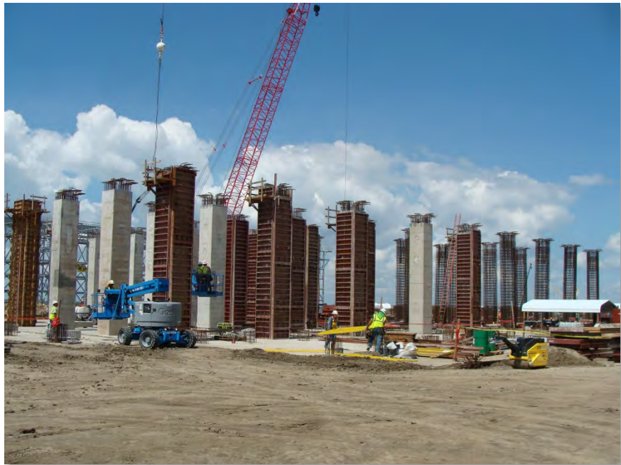
Train 2 132A01 (compressor area columns) (24-Sep-2013)
