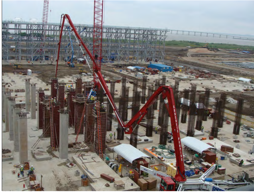
Train 2 (compressor columns) (22-Oct-2013)
