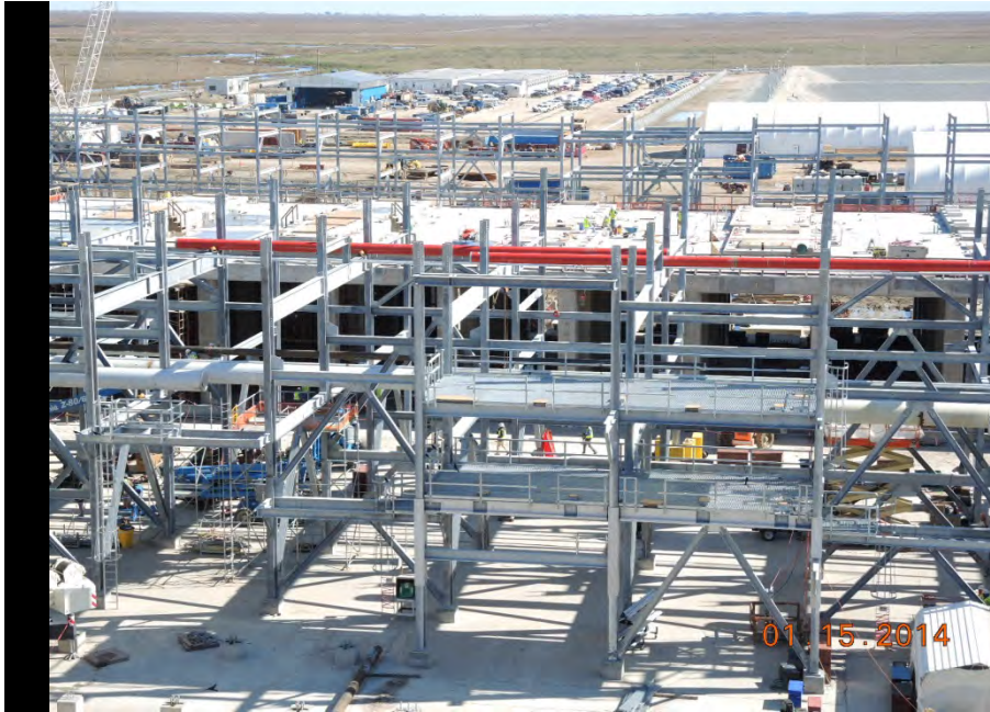
Train 1 131D01 (cryo air coolers piperack) (15-Jan-2014)
