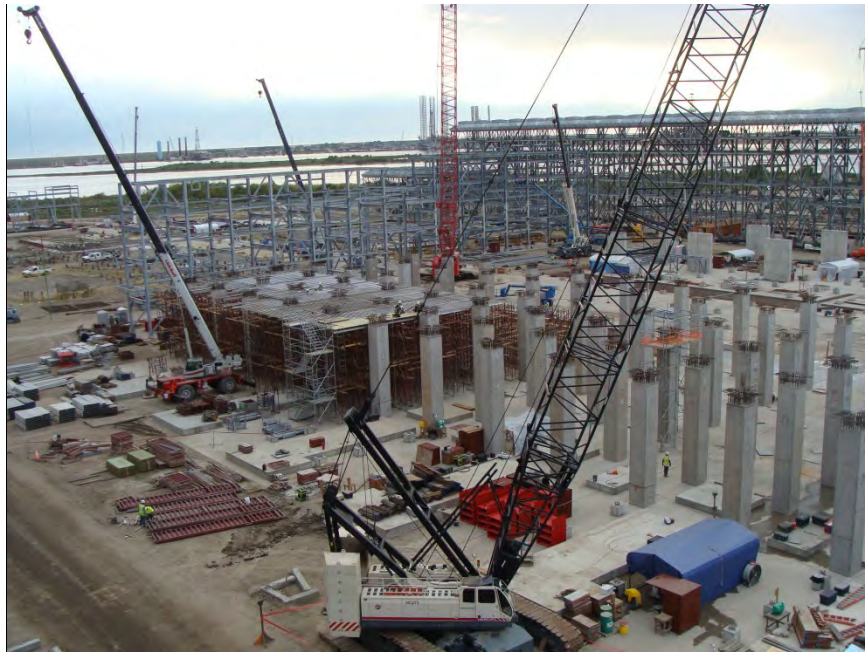
Train 2 (compressor area shoring) (18-Nov-2013)
