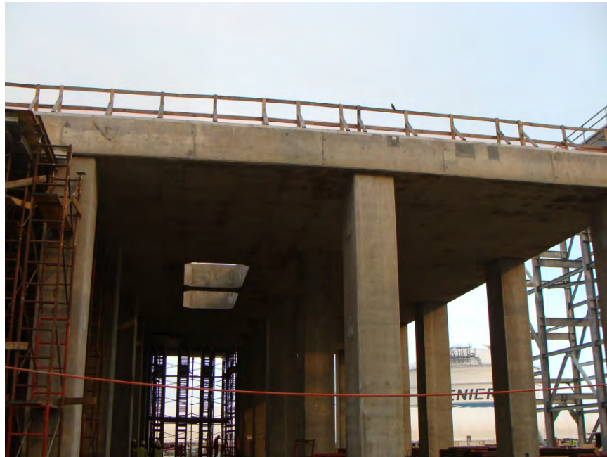
Train 1 (compressor area shoring removal)
