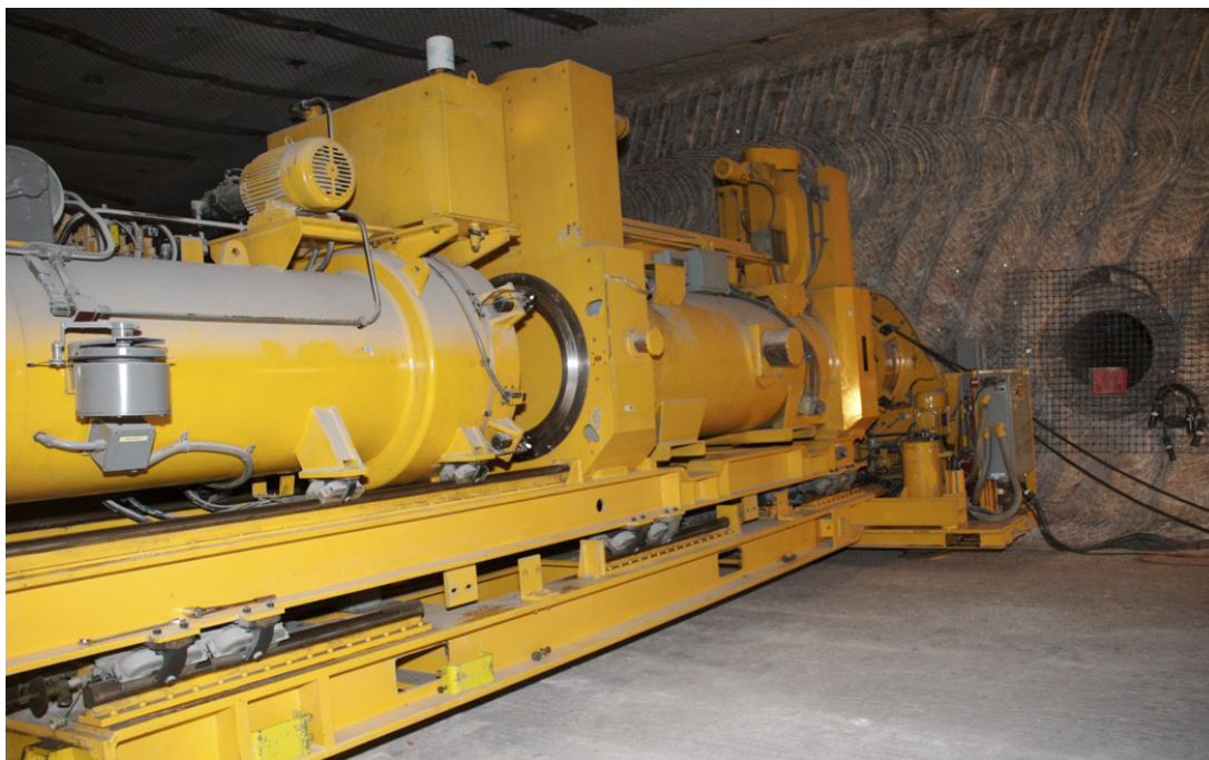
Figure B-10. RH waste disposal equipment used for disposal at WIPP
