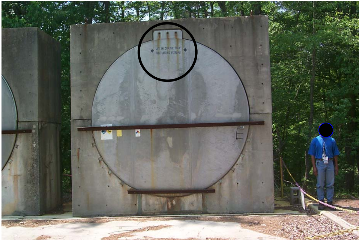
Figure 3-1. Warning Stenciled on the Large Shields
