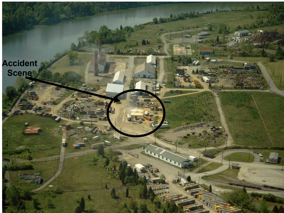
Figure 2-1. Overview of the Accident Scene
