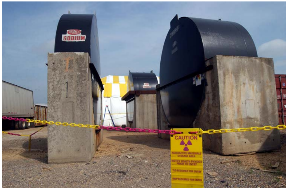
Figure 2-2. Large Sodium Shields
