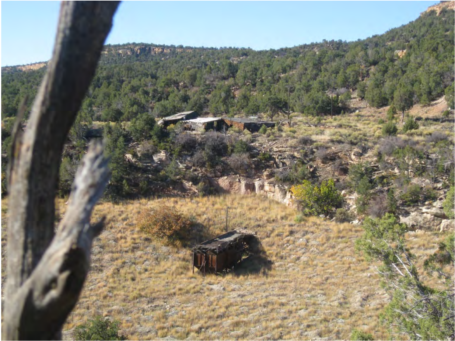
FIGURE 3.12-6 View of the New Verde Mine Reclamation Site on Lease Tract 26 (Remnants of mining structures and an ore bin are present.)
