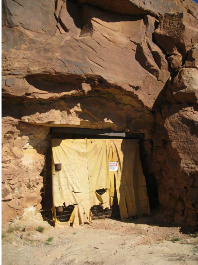
1 2 FIGURE 3.12-8 View of Entrance to Underground 3 Mine at Lease Tract 18 (The Cotter Mine entrance 4 has a locked gate to prevent unauthorized entrance 5 and is covered with fabric to control ventilation.) 6 7
