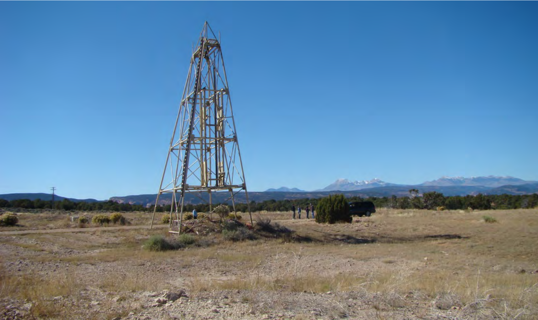
FIGURE 3.12-7 View of Lease Tract 19 Facing West (A headframe structure is located above the closed shaft of the Golden Cycle underground mine.)
