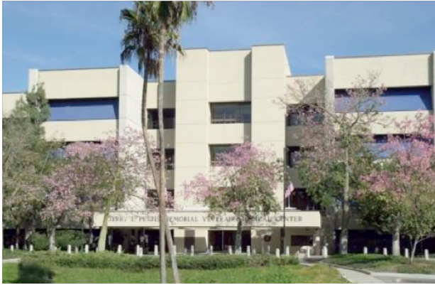
Fuel Cell CHP at the Department of Veterans Affairs: Loma Linda, California http://www.lomalinda.va.gov/images/LLHCSweb.jpg Agency: Department of Veterans Affairs
