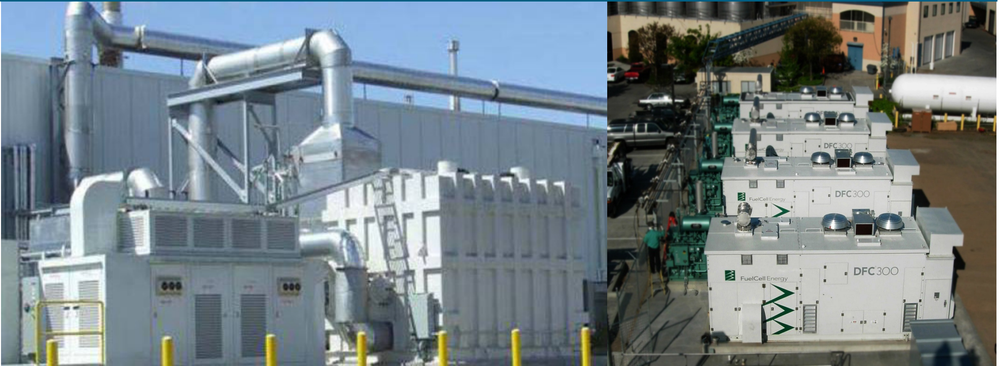
300 kW units: Molten Carbonate Fuel Cell (MCFC), FuelCell Energy, Inc; Fuel Cells Provide Primary Power
