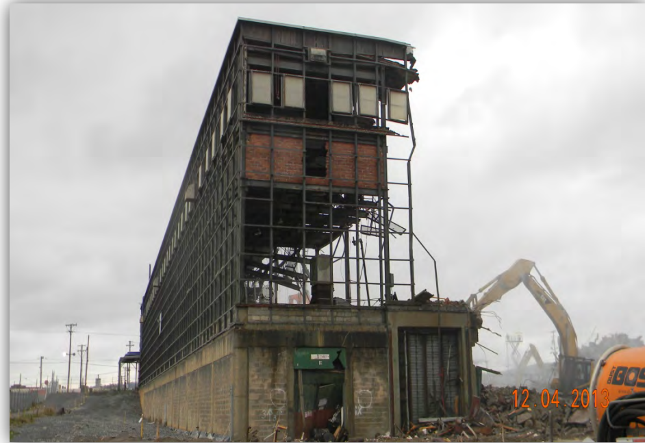
Last of K-25 Building being demolished, Demolition completed Dec. 2013
