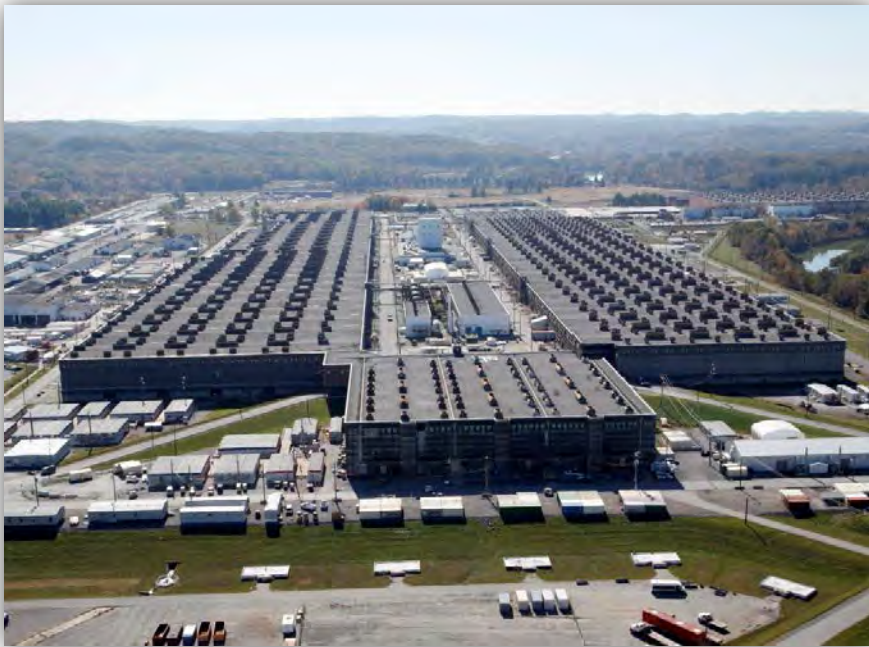
K-25 Building - Before
