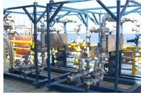
Slip Stream at Wellhead (with BP & Schlumberger)
