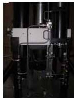
Close-up of piping December 2007
