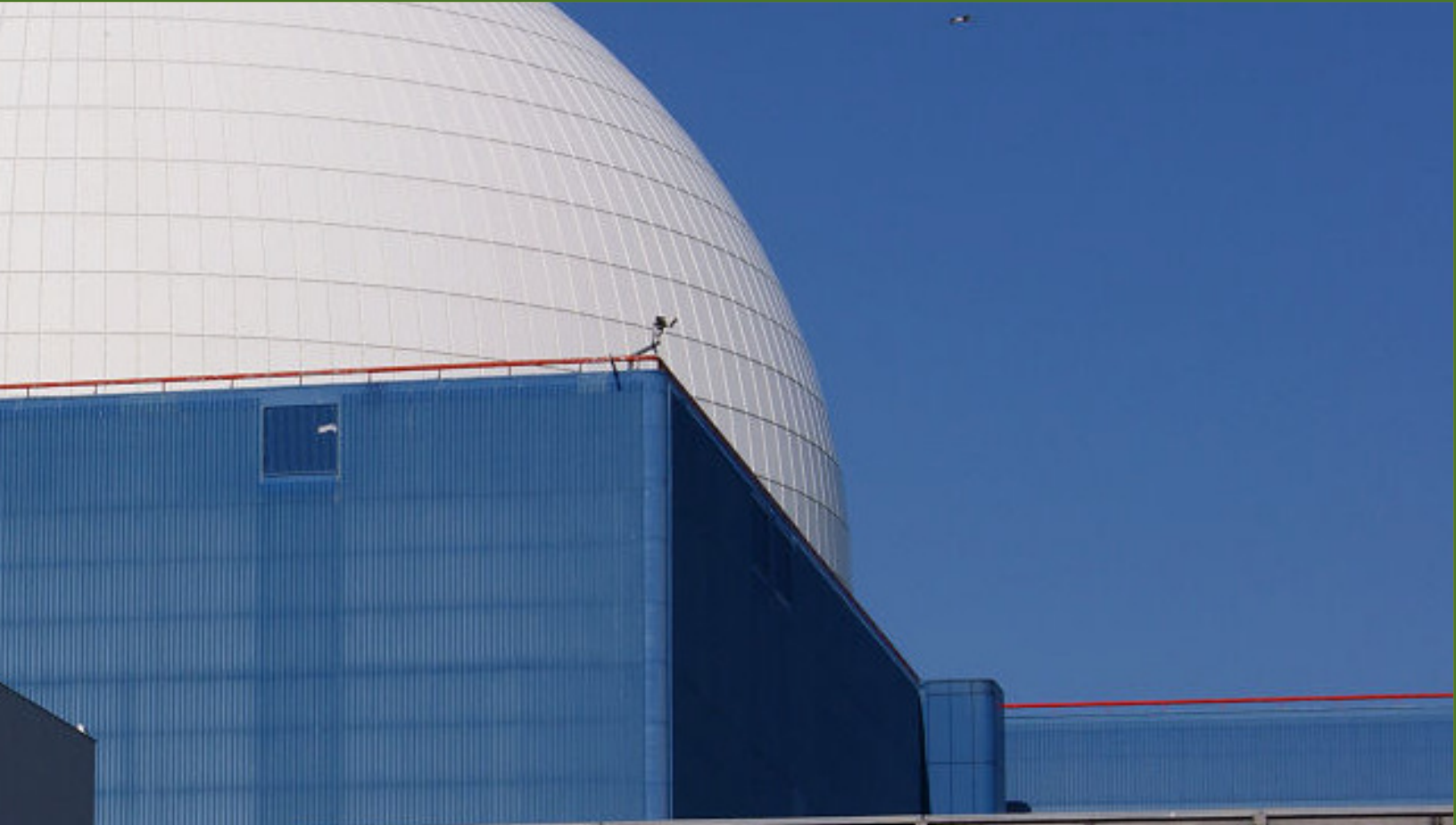
Sizewell Nuclear Power Plant, UK. Photo courtesy of Public Domain
