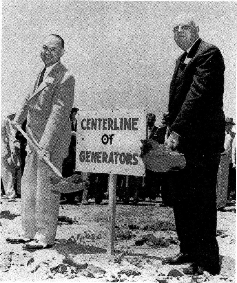
Utility company executives Edgar H. Dixon and Eugene A. Yates break ground in June 1955 for a power plant to supply power for Memphis, Tennessee. The contract between the utilities and the AEC was terminated by President Eisenhower when Memphis officials announced their intention to build a municipal power plant.
