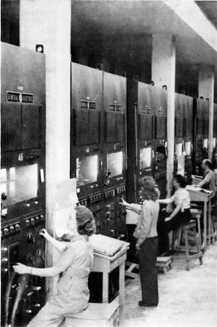
ALPHA I CONTROL ROOM / Each operator tends two control panels, one for each tank. By the spring of 1945, almost 22,000 workers were required to keep Y-12 in operation.
