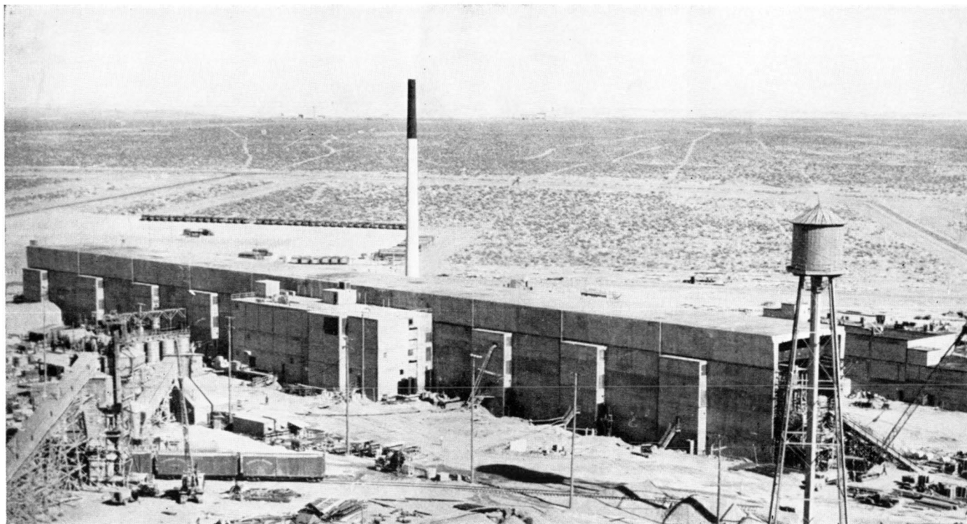
CHEMICAL SEPARATION BUILDING 221-U / The second chemical separation plant nears completion, September, 1944.
