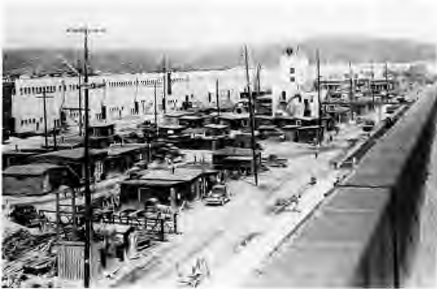
INSIDE THE U AT K-25 DURING CONSTRUCTION / The partially completed gaseous-diffusion plant presented a cluttered appearance in September, 1944.
