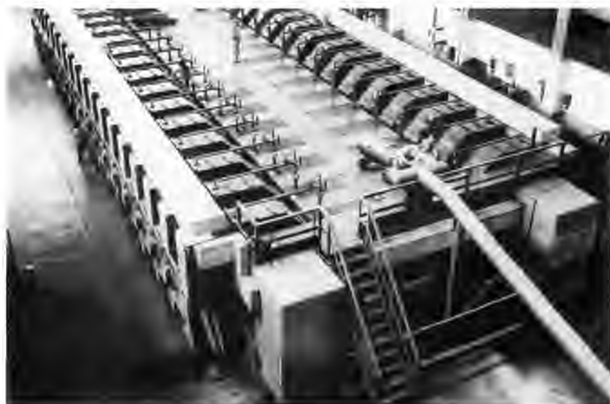
BETA RACETRACK / Compare with the Alpha 1 racetrack, noting the rectilinear arrangement and the smaller scale of the equipment.
