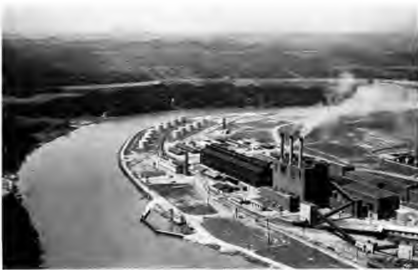
K-25 POWERHOUSE AND S-50 / The power plant (rated capacity: 238,000 kilowatts) stands beside the Clinch River. Behind the power station is the S-50 complex: the main process building, the supplementary boiler plant, and the fuel-oil tank farm.
