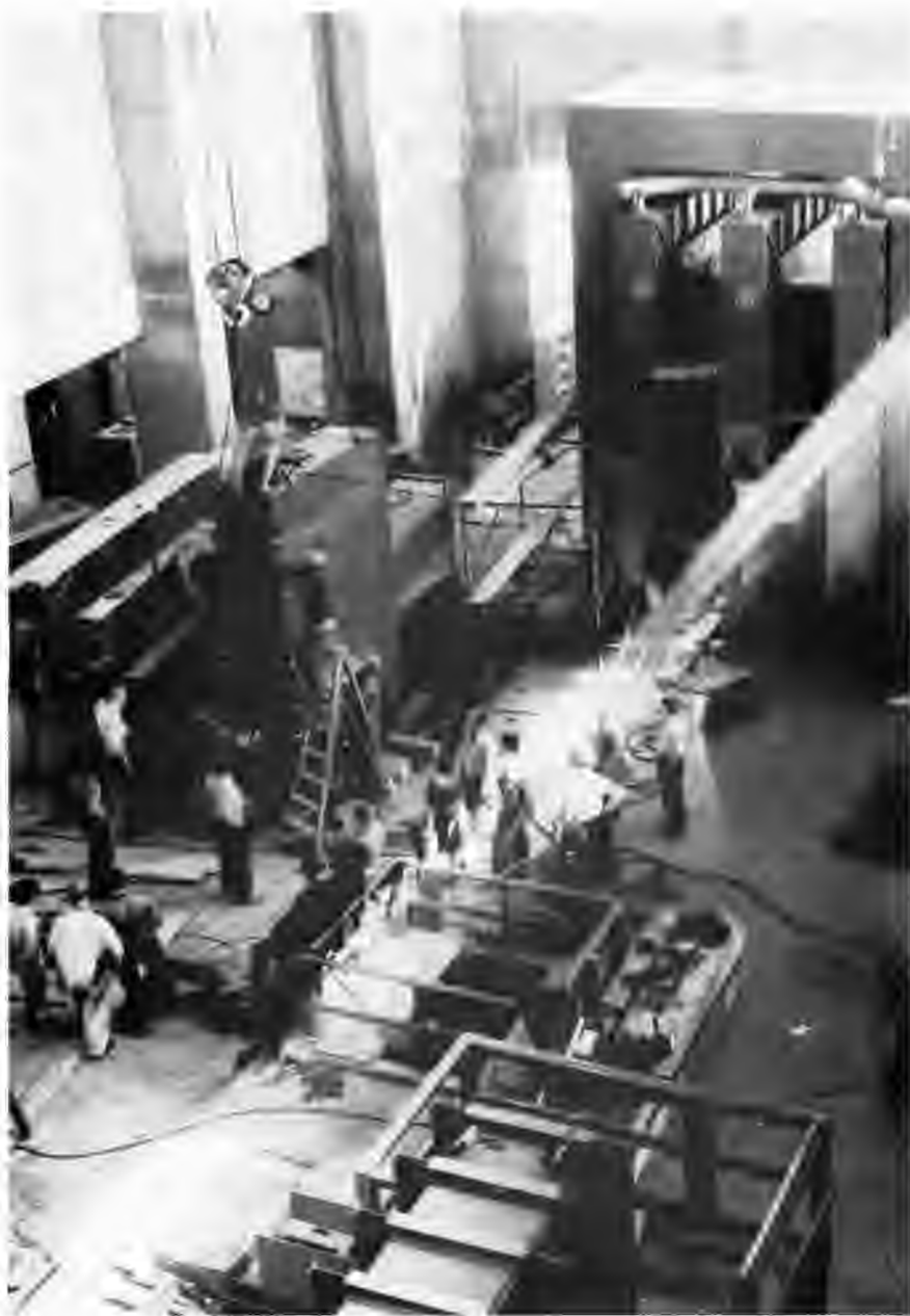
EXPERIMENTAL RACETRACK (XAX) AT Y-12, OAK RIDGE / This unit was built in the summer of 1943 to test the Alpha tracks for the electromagnetic process and to train operators. Workmen are preparing a tank for insertion between the magnet coils.
