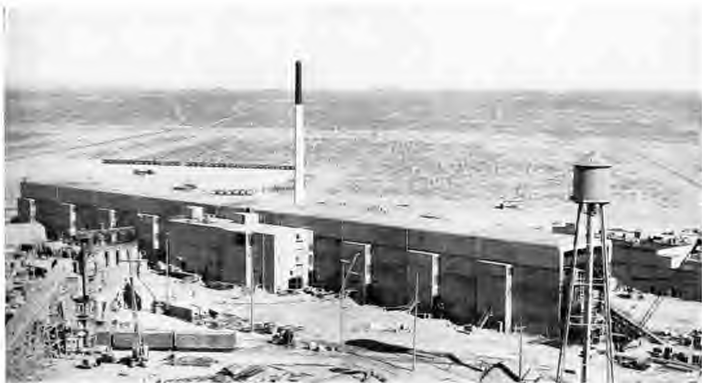
CHEMICAL SEPARATION BUILDING 221-U // The second chemical separation plant nears completion, September, 1944.
