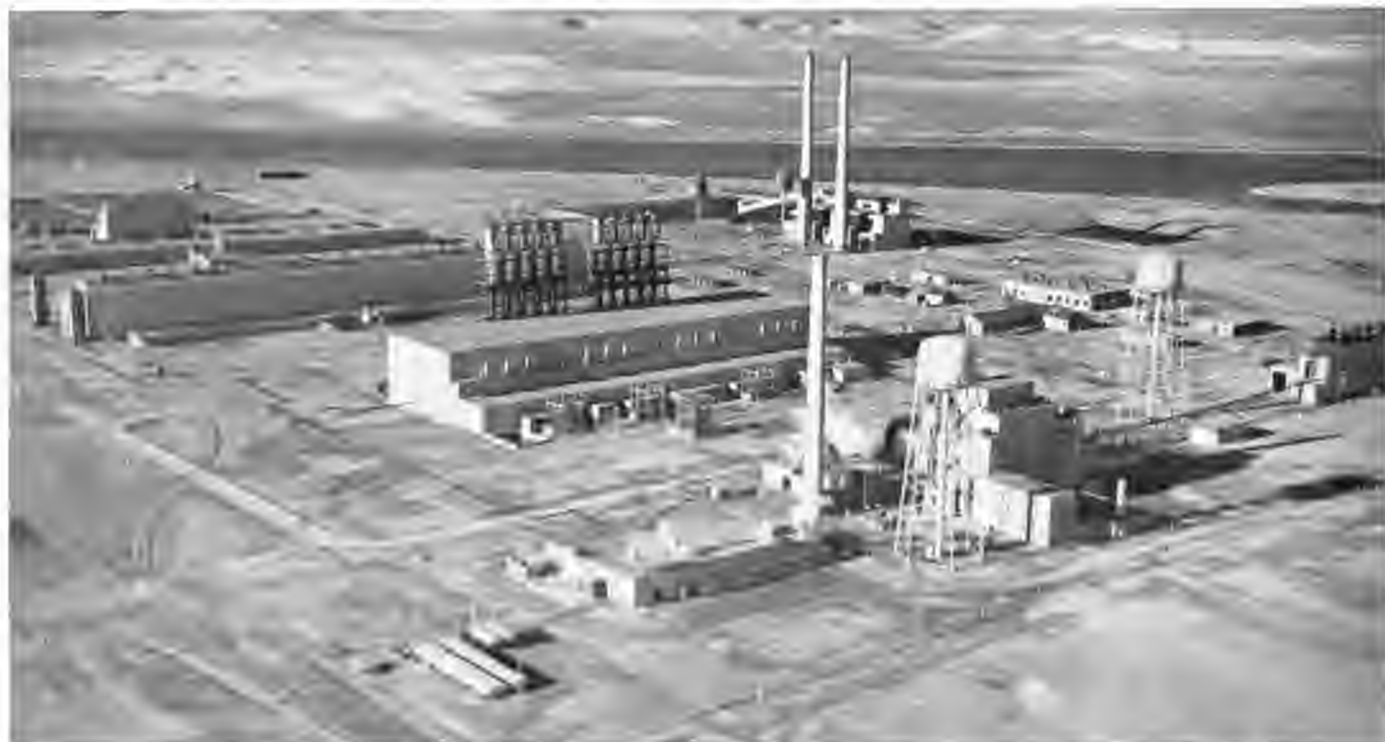
D PILE COMPLETED / This plutonium-production facility at Hanford operated for the first time with 4 full loadings on December 17, 1944.
