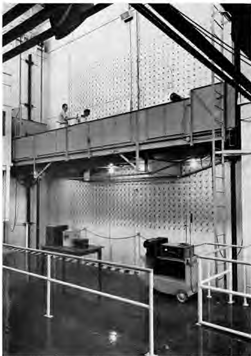
FACE OF THE CLINTON AIR-COOLED EXPERIMENTAL PILE (X-10) / This natural-uranium-and-graphite pile went critical early on the morning of November 4, 1943. Visible on the pile face are the ends of the 1,248 channels in which the uranium slugs are inserted.
