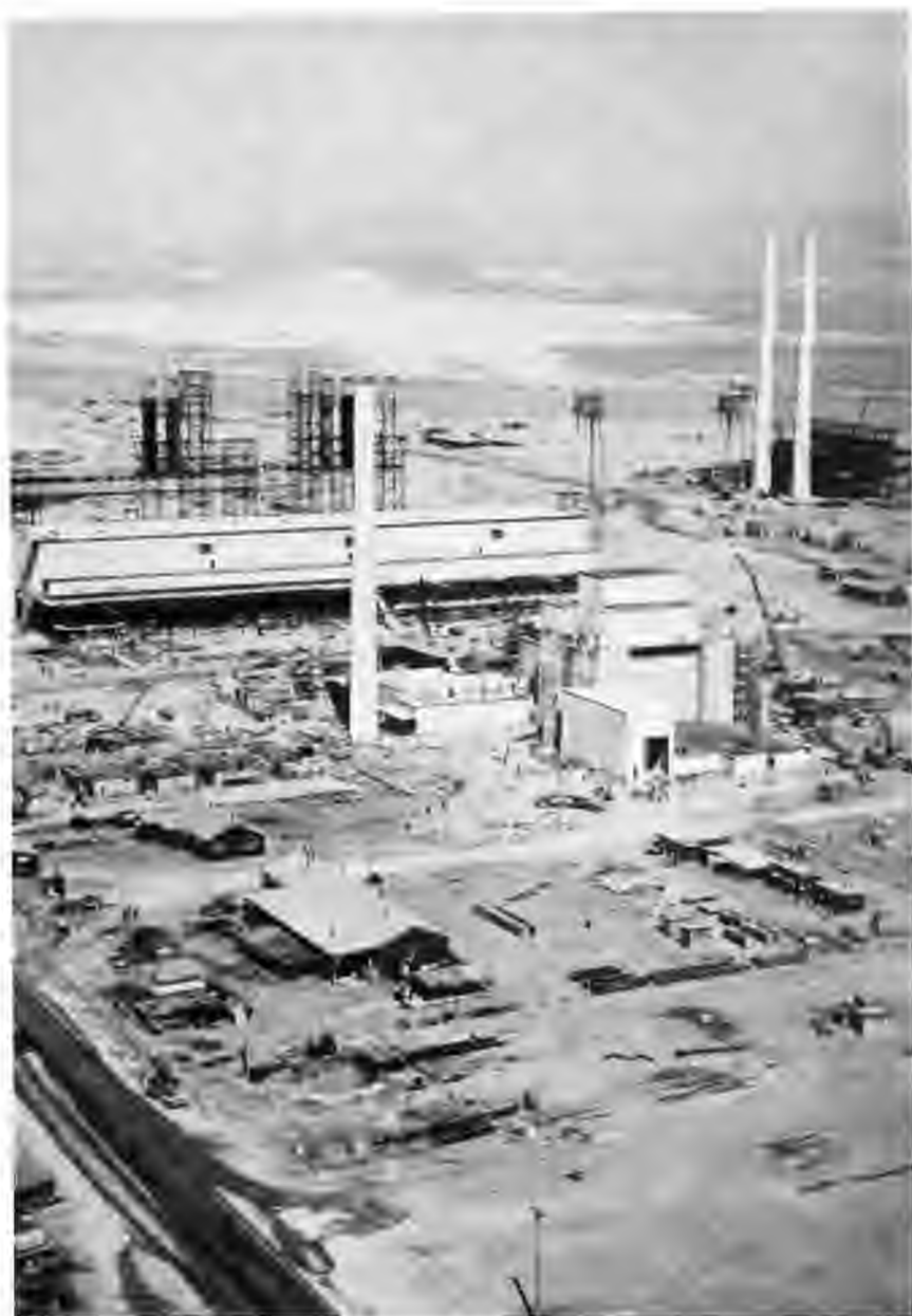
HANFORD D PILE AND SUPPORTING FACILITIES, JUNE 20, 1944 / The pile building, which towered 120 feet above the desert, is the concrete structure in the center. Behind it lies the water-treatment facilities. The Columbia River and the Wahluke Slope are in the background.
