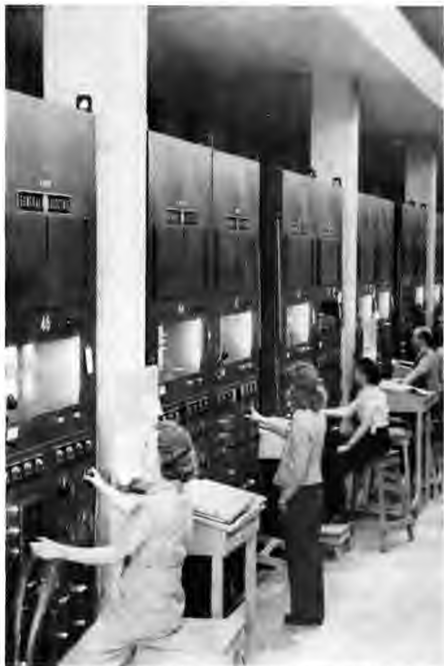
ALPHA I CONTROL ROOM / Each operator tends two control panels, one for each tank. By the spring of 1945, almost 22,000 workers were required to keep Y-12 in operation.
