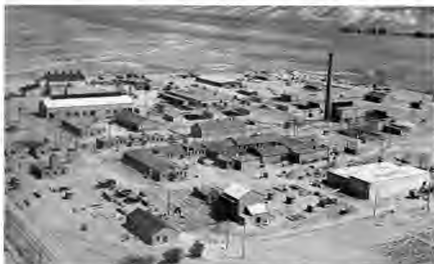
300 AREA AT HANFORD / Here du Pont manufactured uranium slugs and tested materials for the production piles. Slugs were fabricated in the one-story masonry building in the center background. Materials were tested in a 30-watt pile in the large vented building at the upper left.
