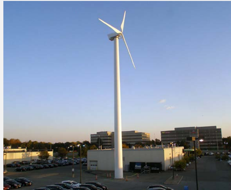
Photo from Byers and Renier Construction, NREL 18221
