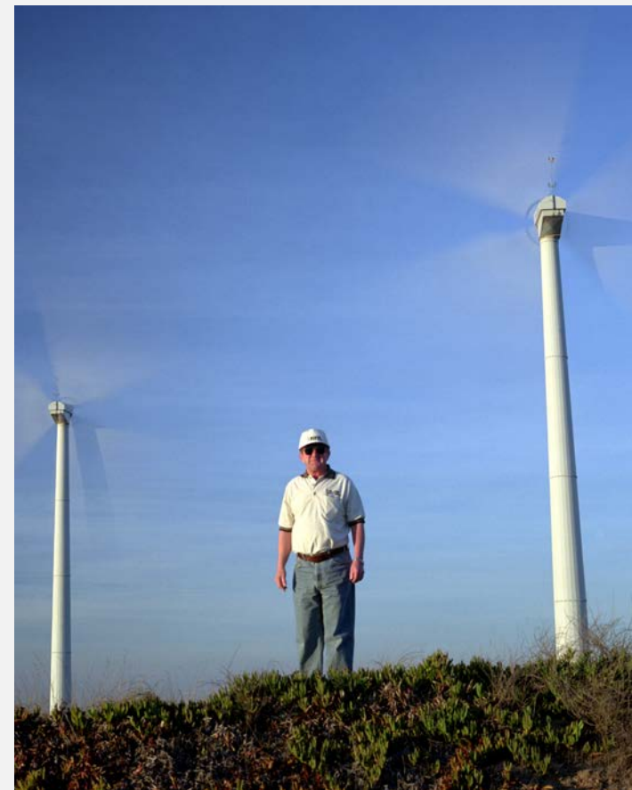
Photo by Warren Gretz, NREL 08684
