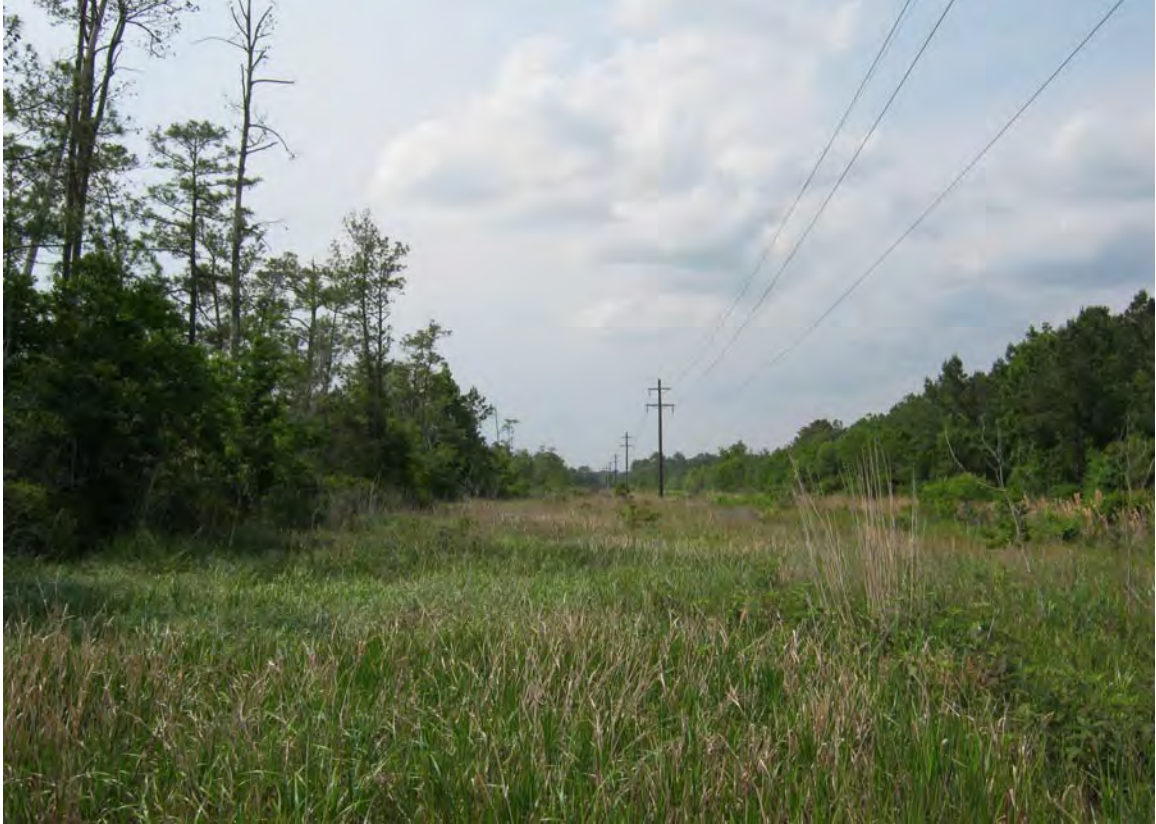
Figure 19. North view of transmission line ROW north of Bayou d'Inde Road.
