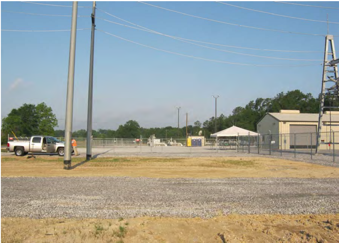
Figure 6. West view of north terminus of pipeline at proposed meter station tie-in.
