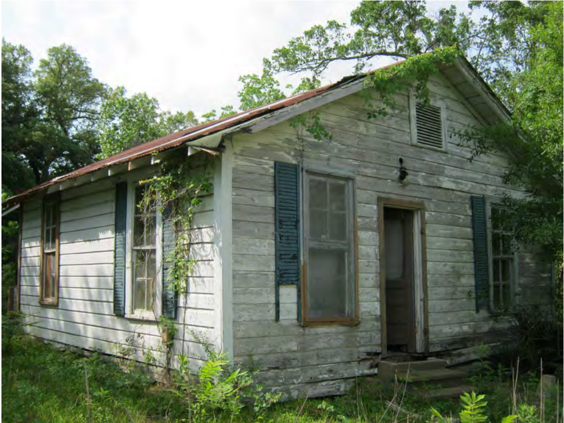
Figure 26. East view of abandoned house on Bayou d'Inde Pass Road near 16CU73.
