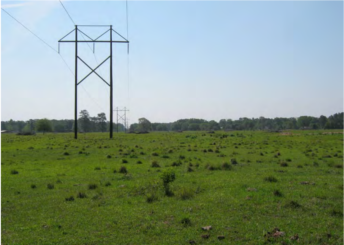
Figure 9. South view of transmission line ROW alignment.
