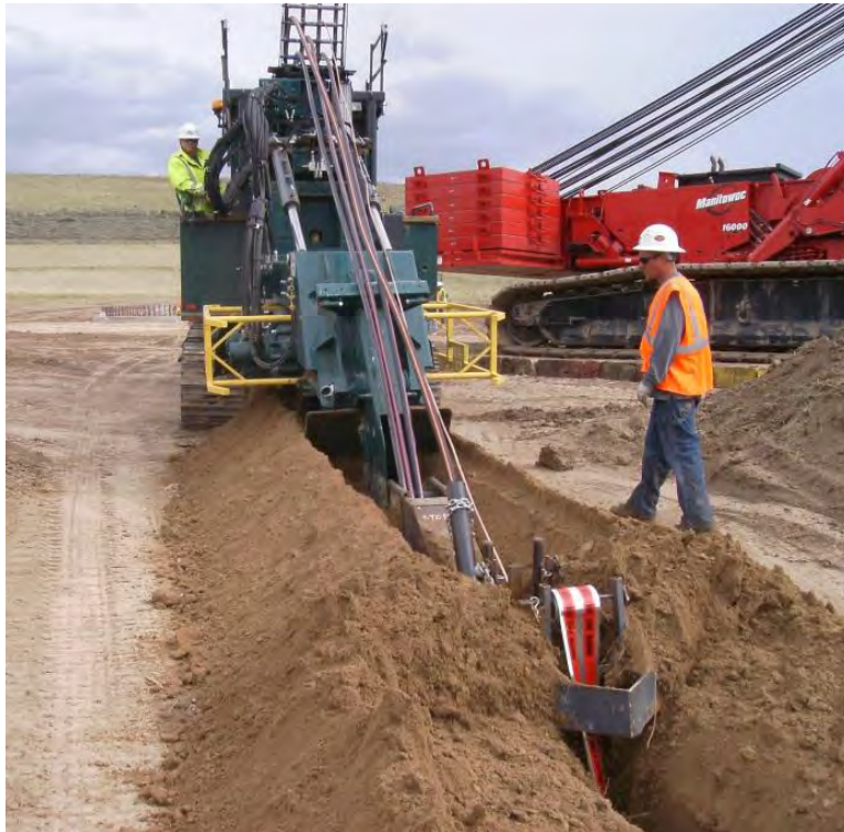
Figure 2-7 Typical Trench for Electrical Collection Cables
