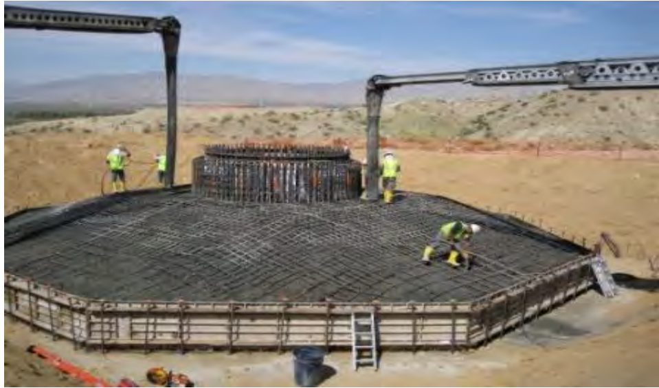
Figure 2-5 Typical Pouring of Turbine Foundation
