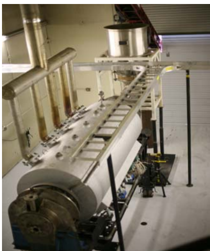
Front End: Feed, Kiln and Burner System
