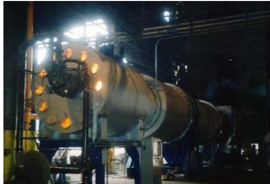
Standard American Oil Co.'s Pyrolytic Hydrocarbon Reactor
