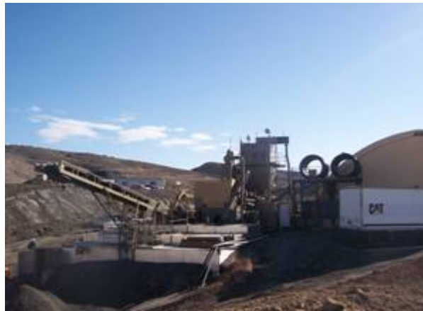
The TME Operational Oil Sands Pilot Plant (100 tph)
