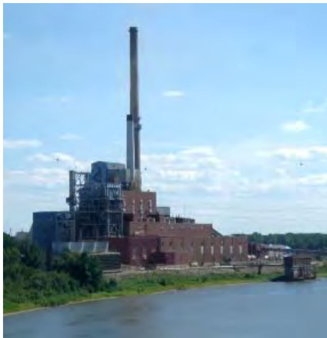
Figure 2-3. Meredosia Energy Center
