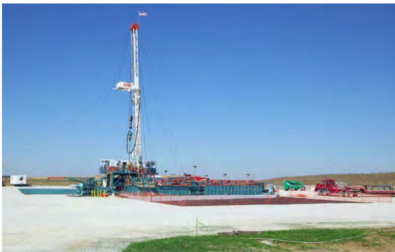
Figure 2-24. Drill Rig during Daytime Operations
