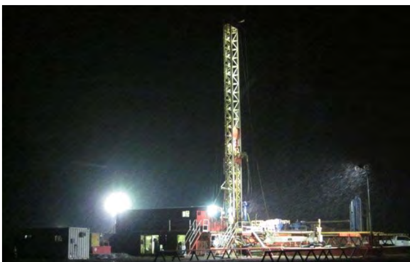
Figure 2-25. Drill Rig during Nighttime Operations
