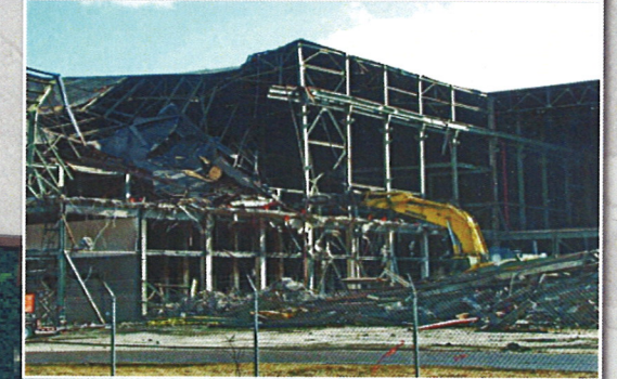
Process Building D&D
