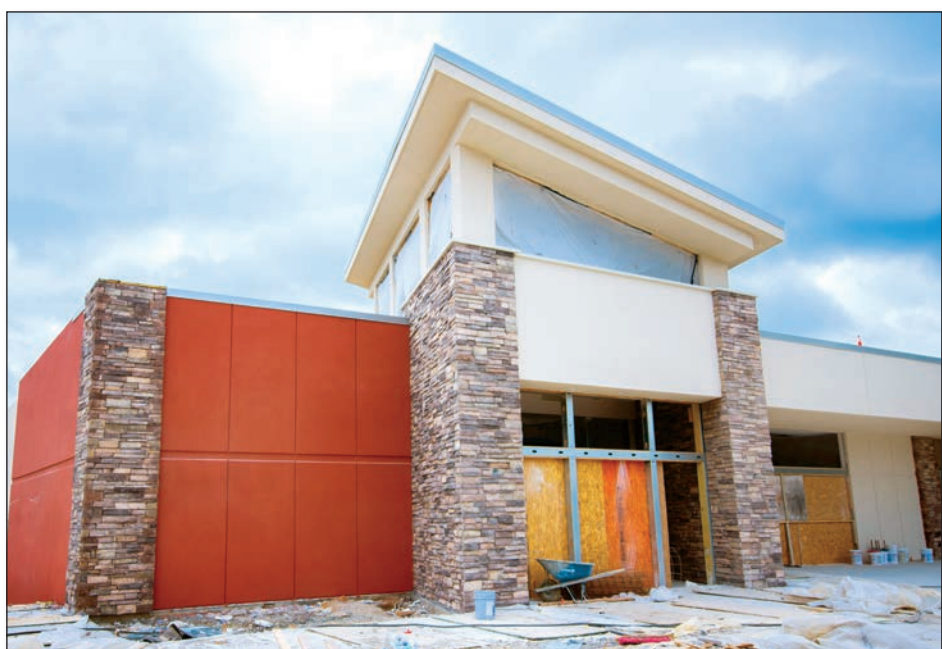
Construction continues on the AMSE entrance in June 2018
