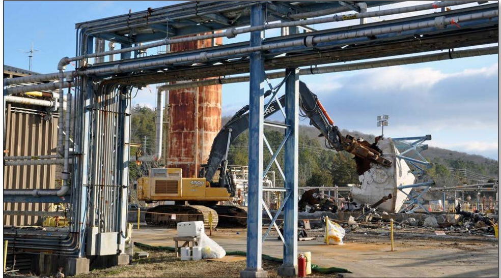
Equipment dismantles piping at the Central Neutralization Facility.
