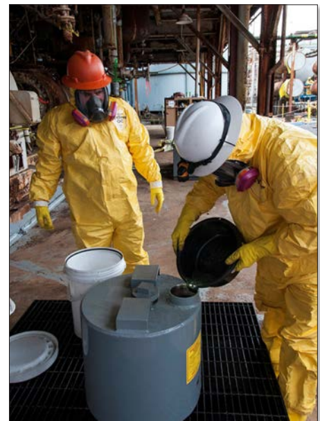
Workers at Y-12 have removed several tons of mercury from equipment at Alpha 4. The drum shown is designed to hold 1,000 pounds of the element.
