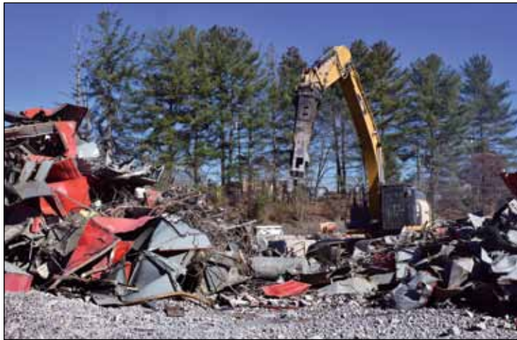
Reindustrialization gains momentum at ETTP with the demolition of Building K-731.
