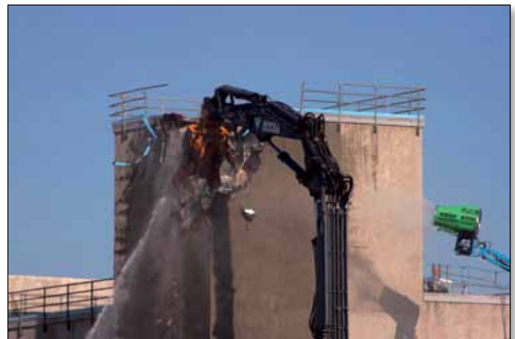
Demolition began at Hanford's Plutonium Finishing Plant in November.
