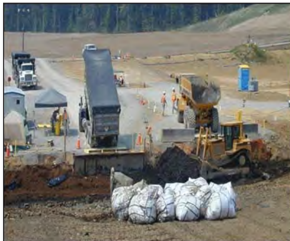
EMWME began receiving waste in May 2002.
