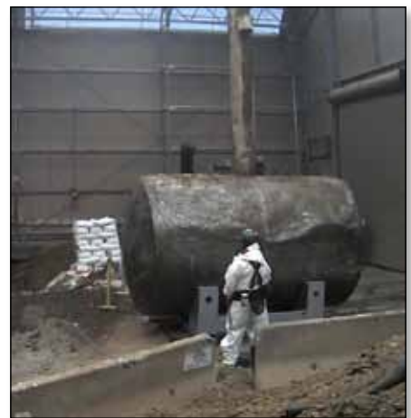
Tank W-1A following excavation.
