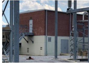
Type 2: Concrete With Steel Rebar
