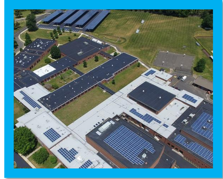
Energy & Frequency Regulation from Solar-Storage Microgrid
