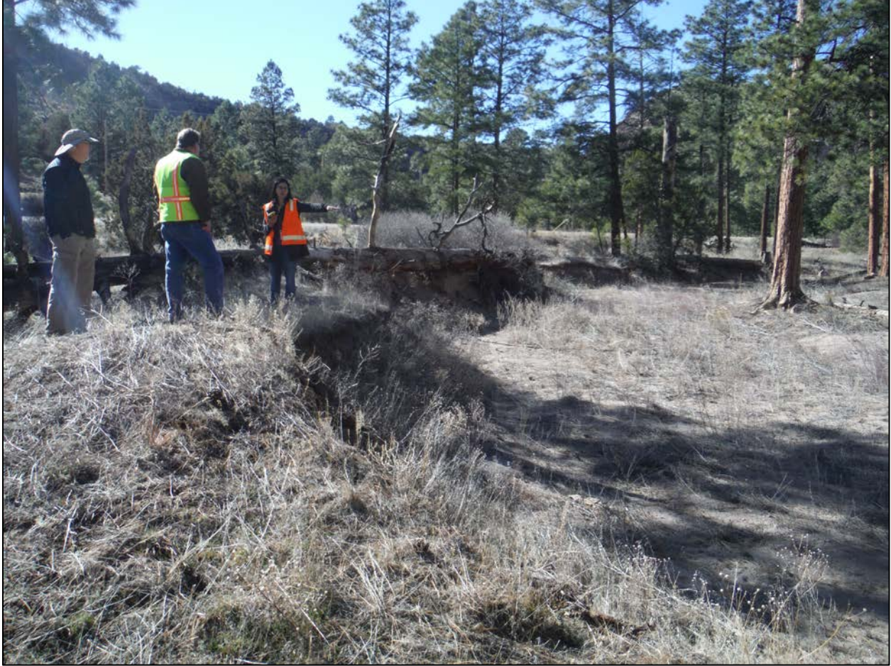
Photograph 3. An unstable bank in the lower project site
