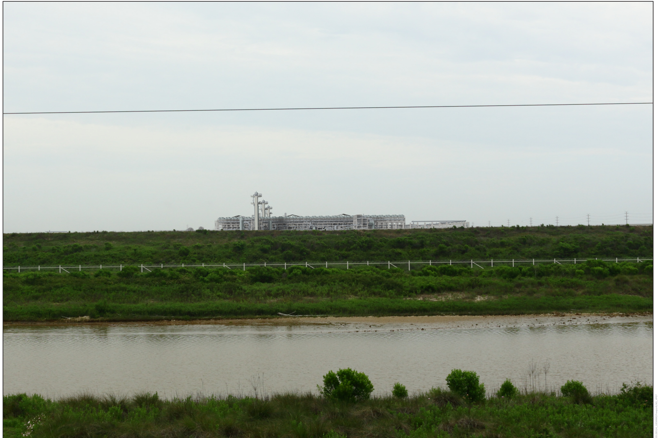
Figure E-4 Northern end of 806c - Looking North East - Proposed View (Ground Level) Enlargement Area of Figure E-3
