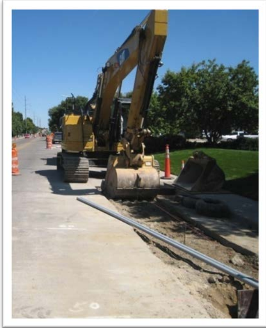
230-kV duct bank under construction, Longmont, Colorado
