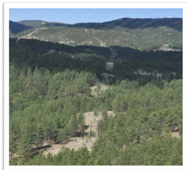
Photograph from a helicopter traversing the Southern Rocky Mountains. Vegetation management and the dissected terrain allows for mature trees to grow under the transmission lines in ravines and other low points.
