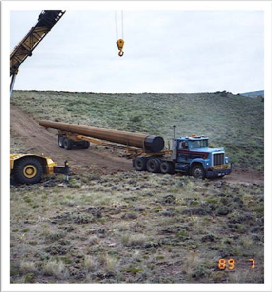
Hauling structure on an access road
