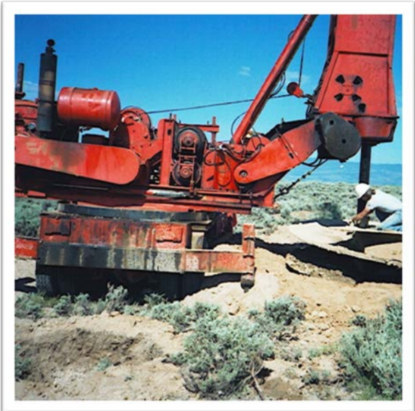
Auger drilling for structure base
