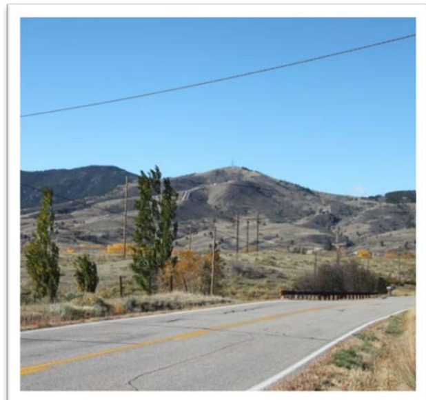
Photograph from County Road 18E north of Flatiron Reservoir of Bald Mountain, with the penstocks, radio towers and several electrical transmission and distribution lines including the E-LS and F-PH lines.
