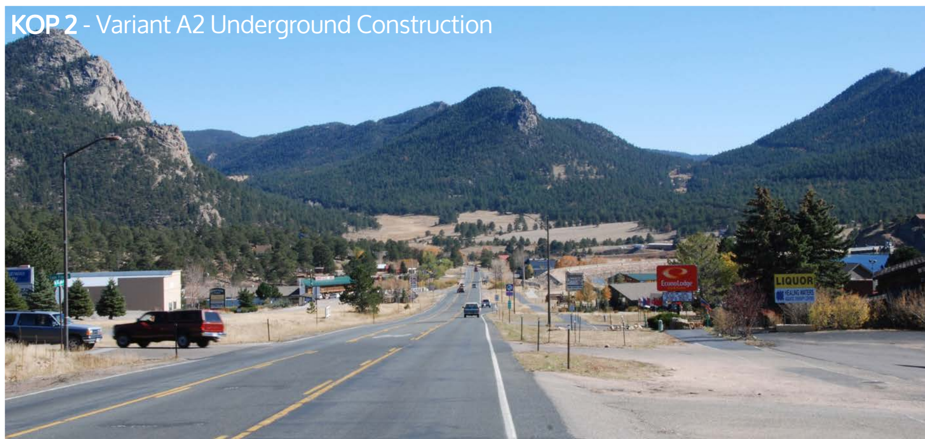
Underground construction of Double Circuit Line on a Consolidated ROW with Re-Routes
