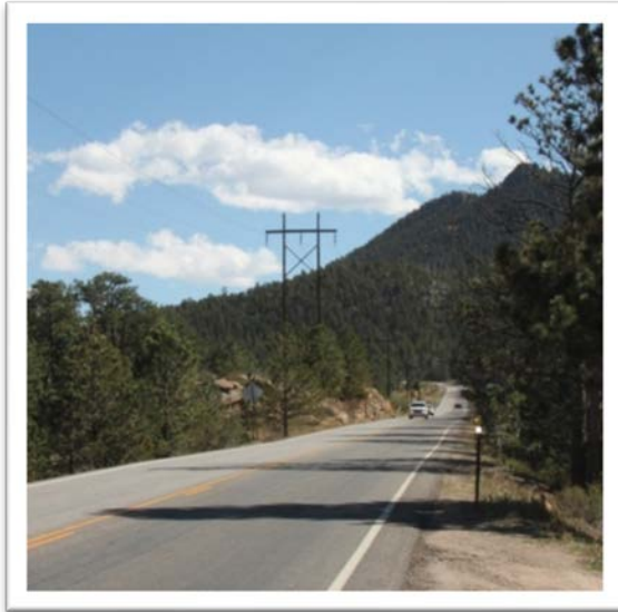
Photograph of E-PH transmission line along U.S. Highway 36 approaching leaving Estes Park in the Southern Rocky Mountains landscape character unit.
