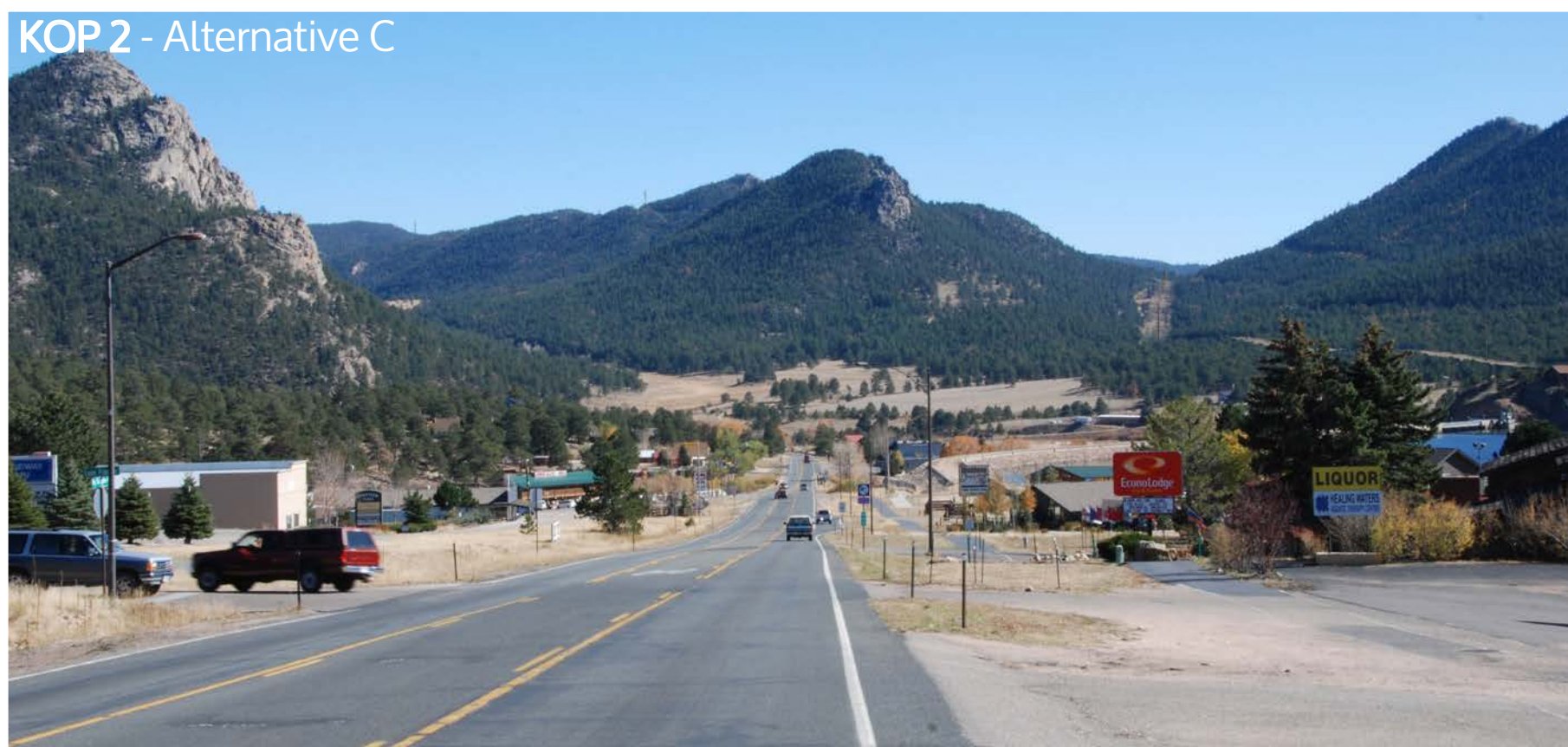
Double Circuit Line on a Consolidated ROW Using North and South Alignments
