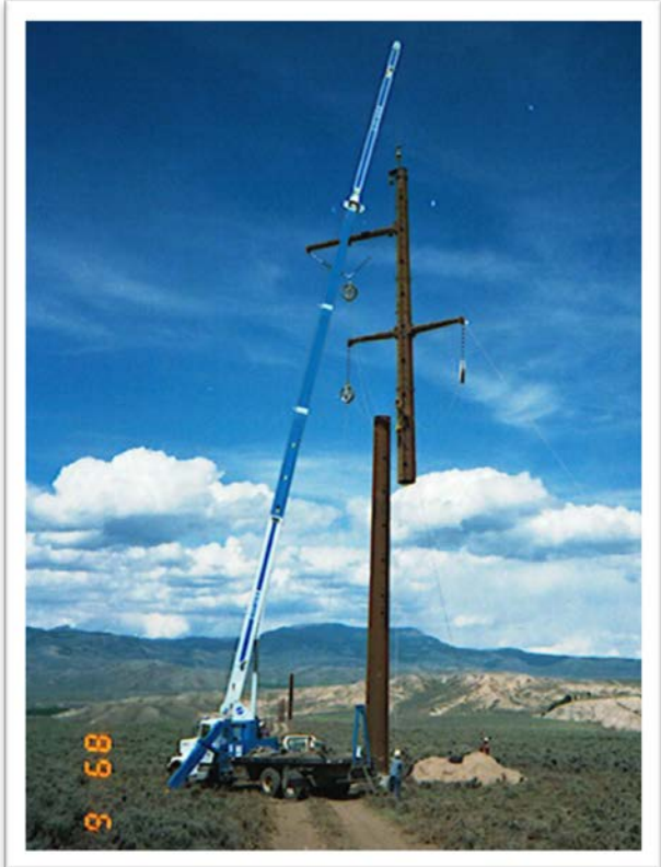
Setting the top of a structure
