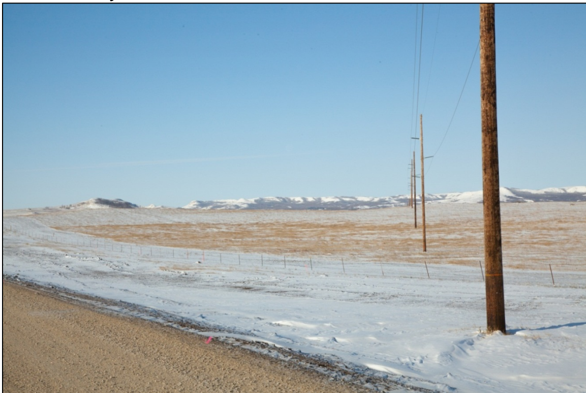
Figure 3-34: 115-kV Transmission Line in the Killdeer Mountain Battlefield Study Area
