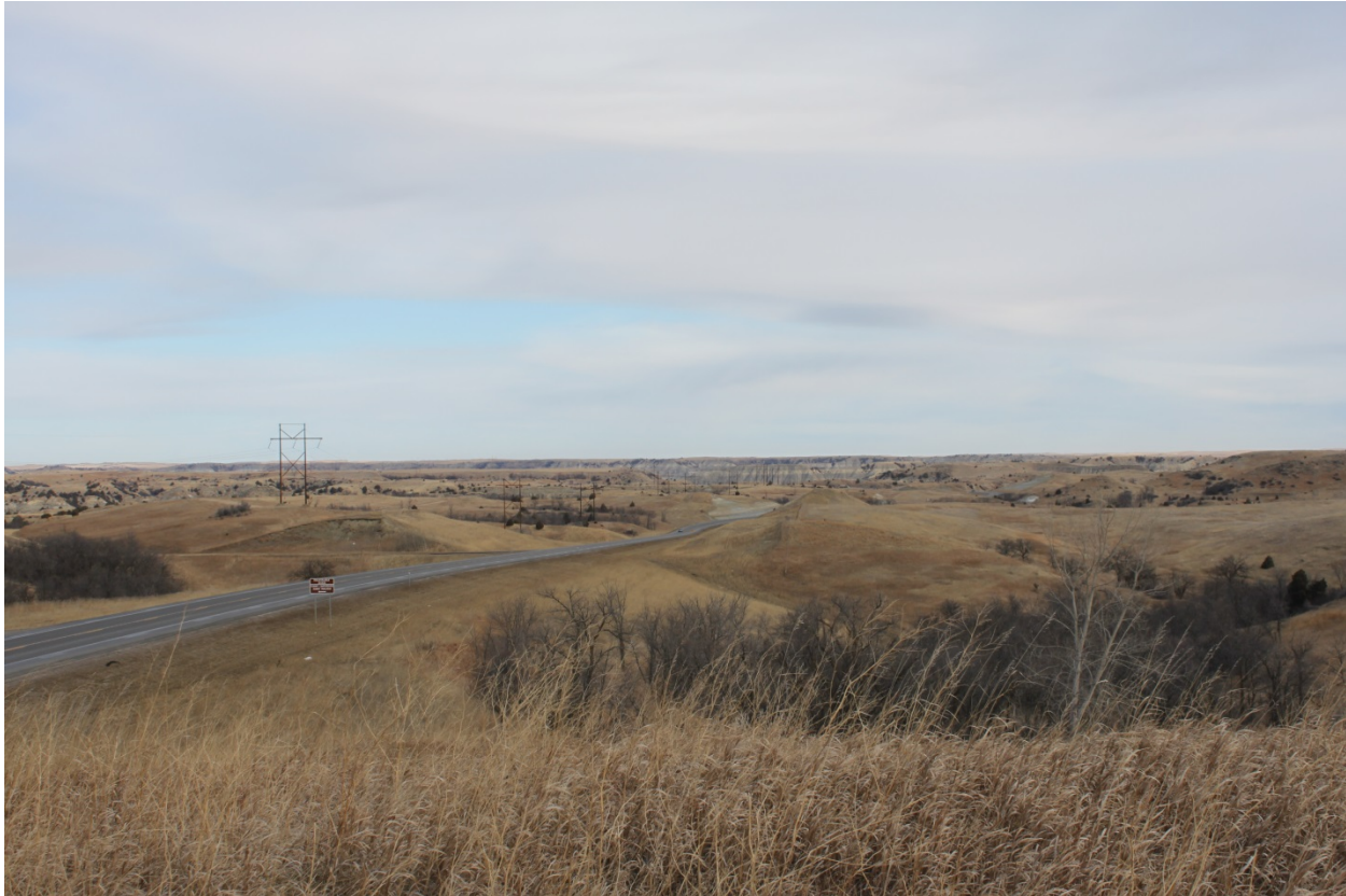
Figure 3-13: Existing Views of U.S. Highway 85 and Western's 230-kV Transmission Line
