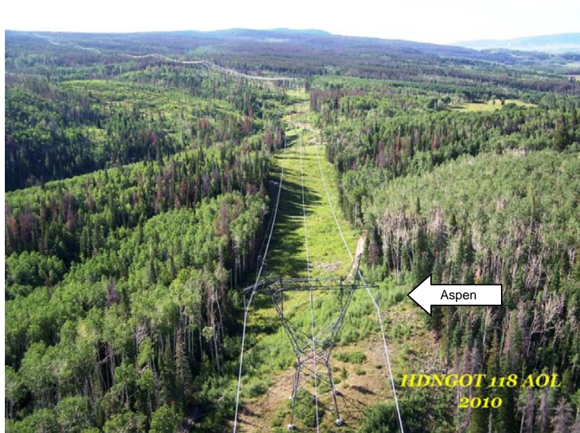
Photo 2-7. The ROW was cut when the line was constructed and has been maintained in a desirable condition. Note that aspen and lodgepole pine are the predominant species, with rapid aspen regeneration occurring immediately behind the first transmission line structure. Western would monitor the ROW and treat it as needed to maintain this condition.
