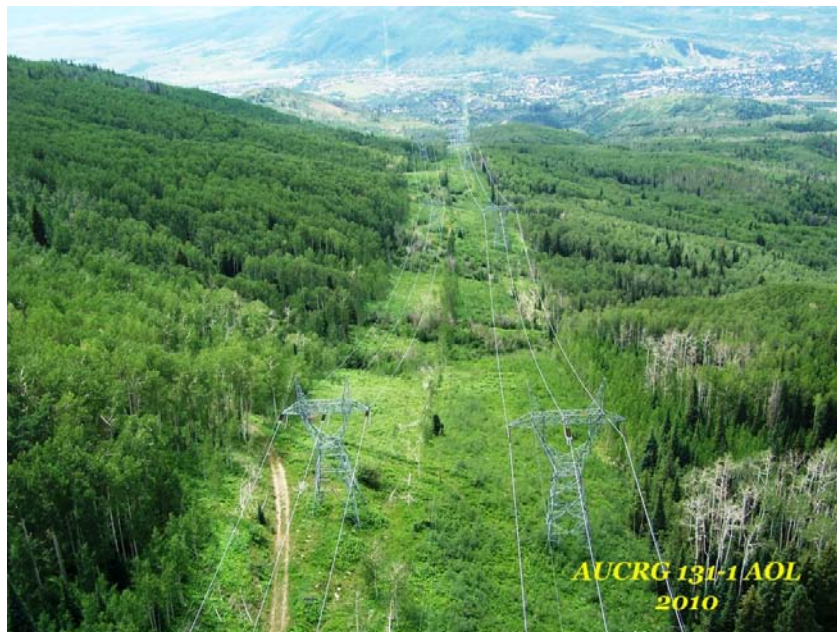
Photo 2-8. These parallel ROWs have been maintained in a desirable condition through a stand of predominantly aspen.
