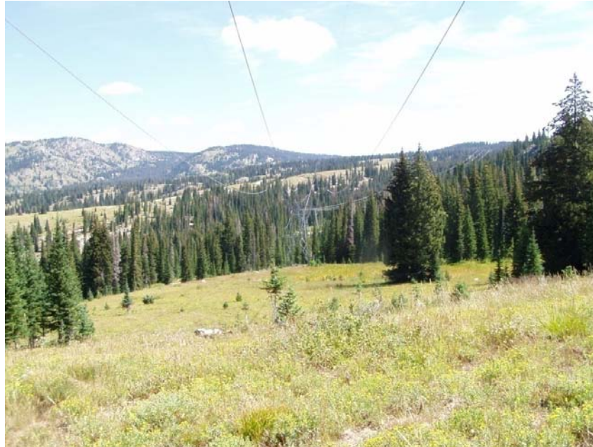
Photo 2-15. Although this ROW is generally acceptable, the two larger trees under the transmission line are due for treatment to ensure they do not present a hazard to the line.
