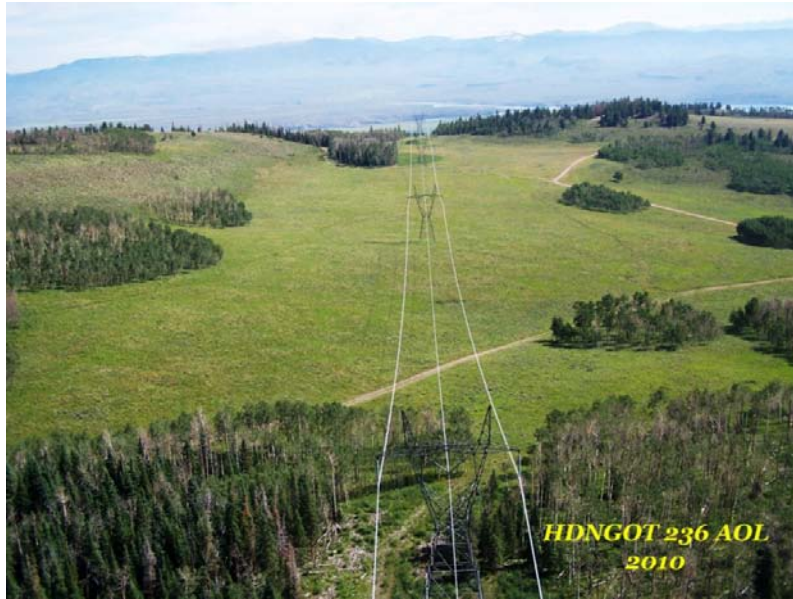
Photo 2-1. ROW with natural, low-growing vegetation outside the aspen stands that is compatible with the transmission line.
