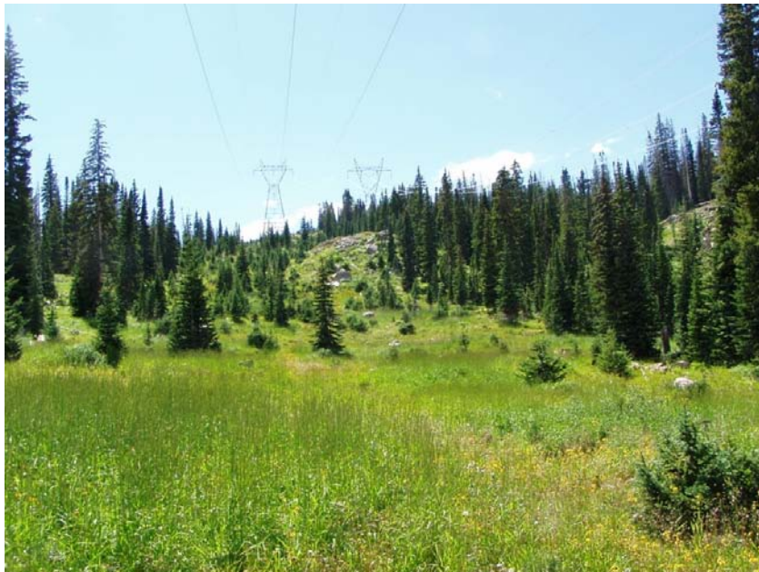
Photo 2-12. These two parallel lines have different authorizations for vegetation maintenance. The line on the left is in a desirable condition, but Western will monitor it and treat as needed. The line on the right is not in a desirable condition; Western would schedule it for initial treatment and then maintain it in a condition similar to the line on the left.
