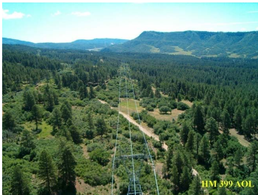
Photo 2-16. Western would monitor potential fuel loading under the lines and near the structures, and schedule treatment as needed.
