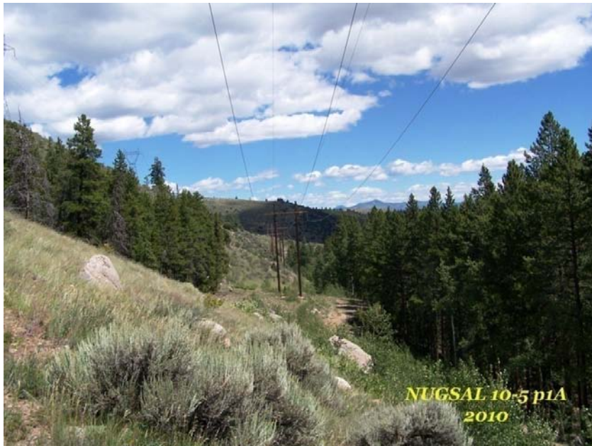
Photo 2-14. The condition of this ROW is generally acceptable and relatively stable, but will require monitoring to ensure that the need for treatment can be identified and implemented. Note the low level of aspen re-growth in the lower right corner, which has emerged and must be closely monitored.
