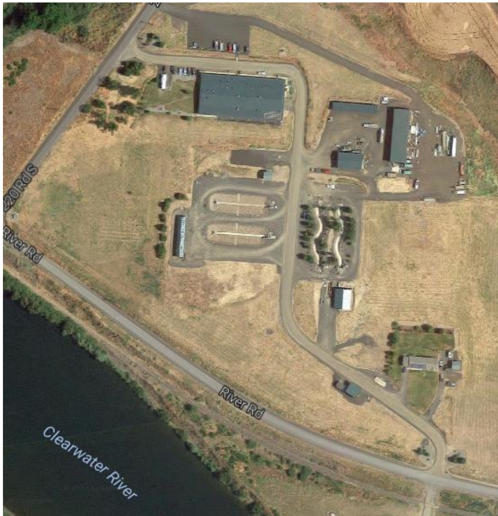
Figure 5 Existing facilities at NPTH
