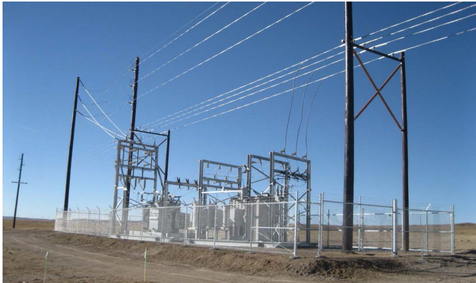
Figure 9. Example of Skid Mounted Substation
