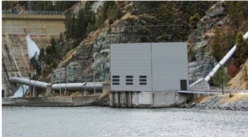
Figure 4. Future Pumping Plant Building Enclosure.
