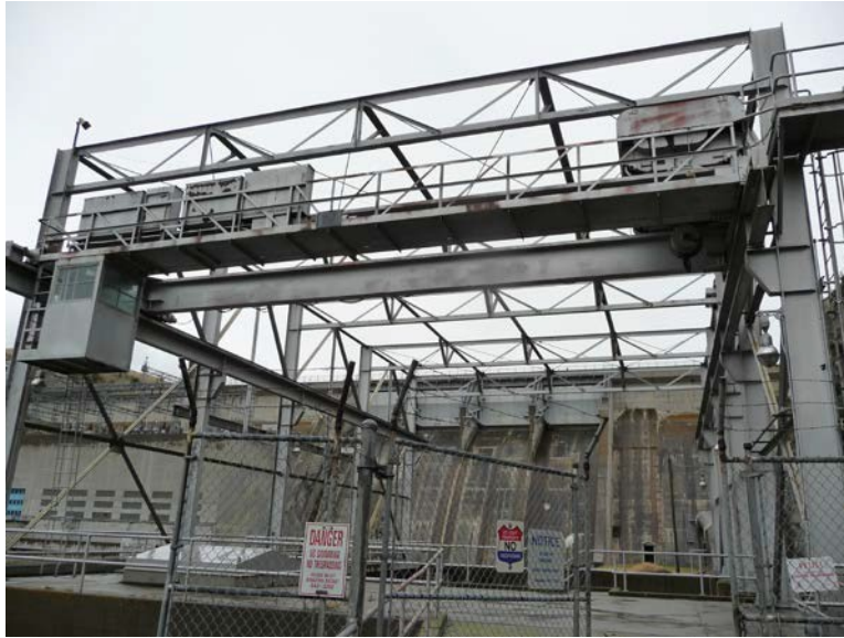
Figure 3. Existing Pumping Plant.
