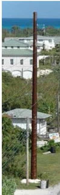
Figure 8. Typical weathered pole.
