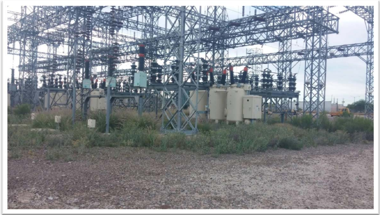
Figure 1-4 Vegetation at Tucson Substation
