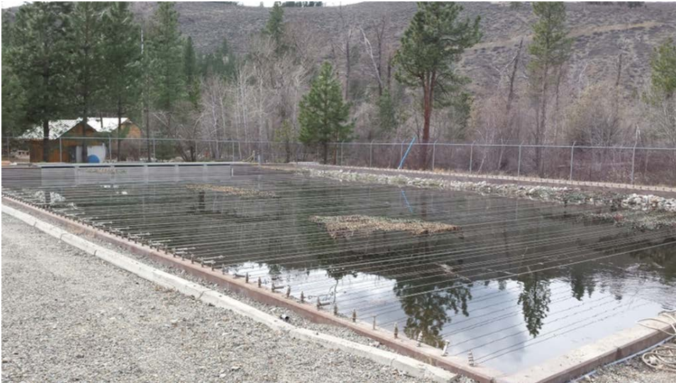
Figure A-1. Chewuch Acclimation Facility
