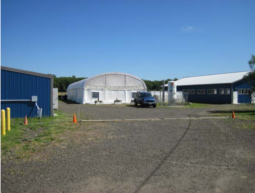
Photograph 1 – Overview of Burley Creek Hatchery in Port Orchard, Washington (view looking north).
