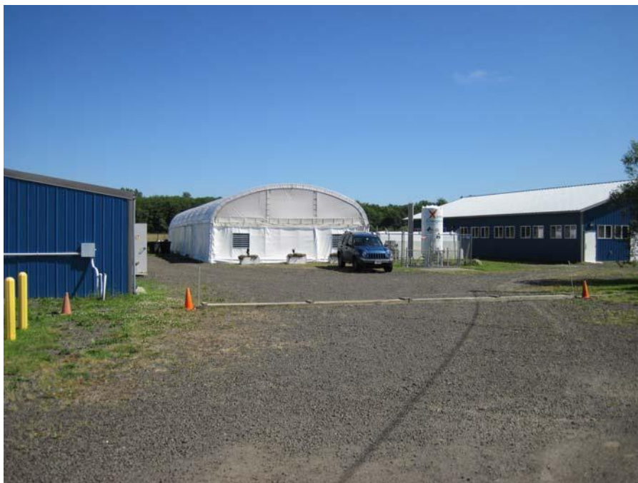
Photograph 1 – Overview of Burley Creek Hatchery in Port Orchard, Washington (view looking north).
