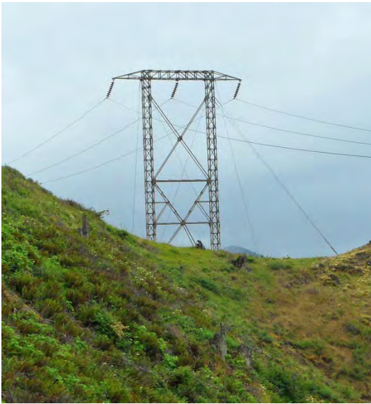
Figure 2.1-2. Photos of Existing Lattice-steel H-frame and Wood-Pole H-frame Structures along the Bonneville-Hood River Line
