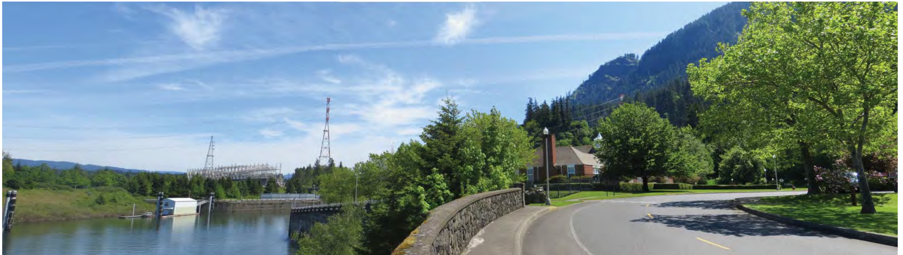
Figure C-2. Project Area Right-of-Way is Visible to the East in Center of Photo Viewed from the Bonneville Dam Visitor Area KVA
