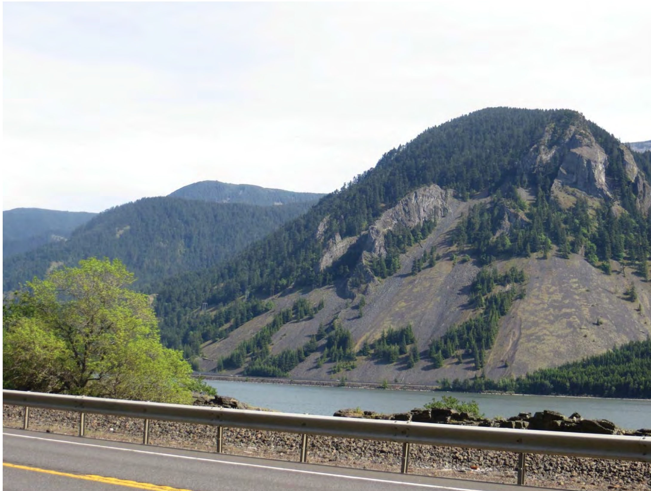
Figure C-6. Steel Structures are Visually Evident along Talus Slopes of Shellrock Mountain (lower left of photo) as seen from the SR 14 KVA when Looking South
