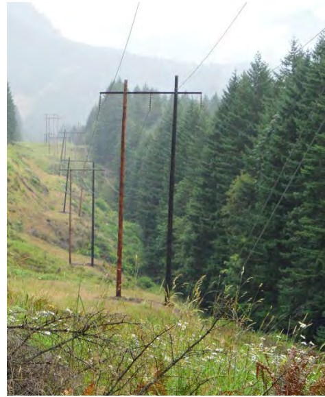
Figure 2.1-2. Photos of Existing Lattice-steel H-frame and Wood-Pole H-frame Structures along the Bonneville-Hood River Line
