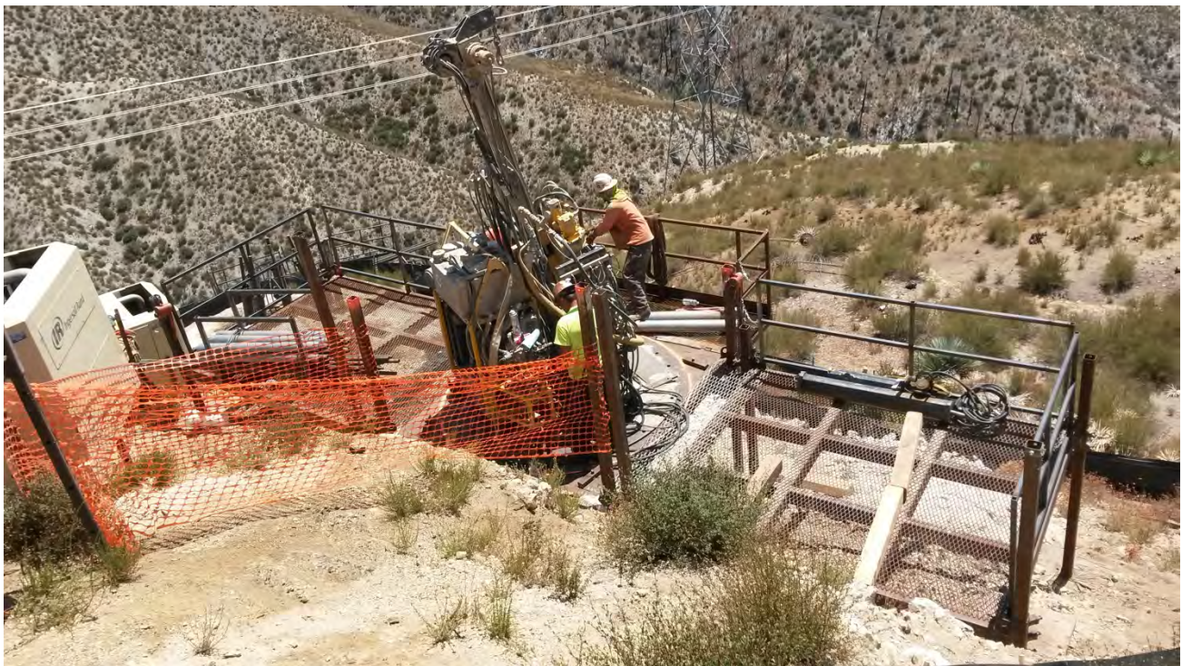
Figure 2.1-7. Example of Temporary Mobile Work Surfaces and Micropile Drill Rig
