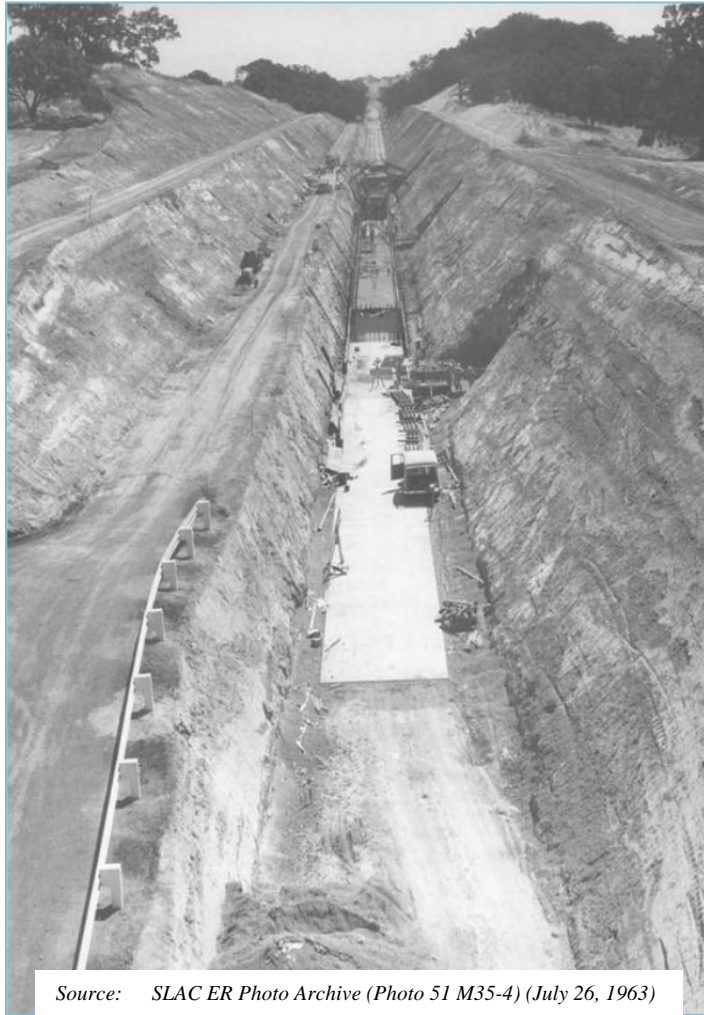
Figure 3-2 View of Excavation for Accelerator Housing Looking East from Sector 0
