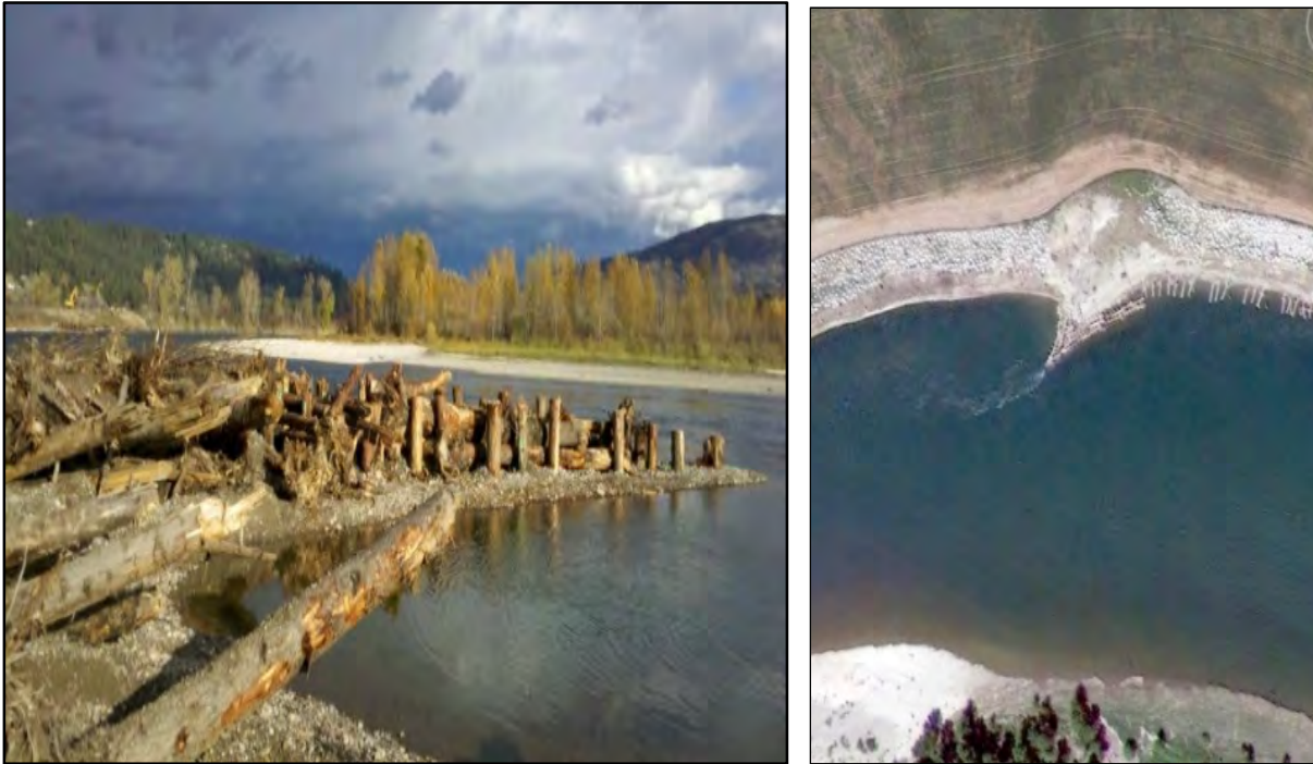
Figure 2-3. Examples of Pool-forming Structures
