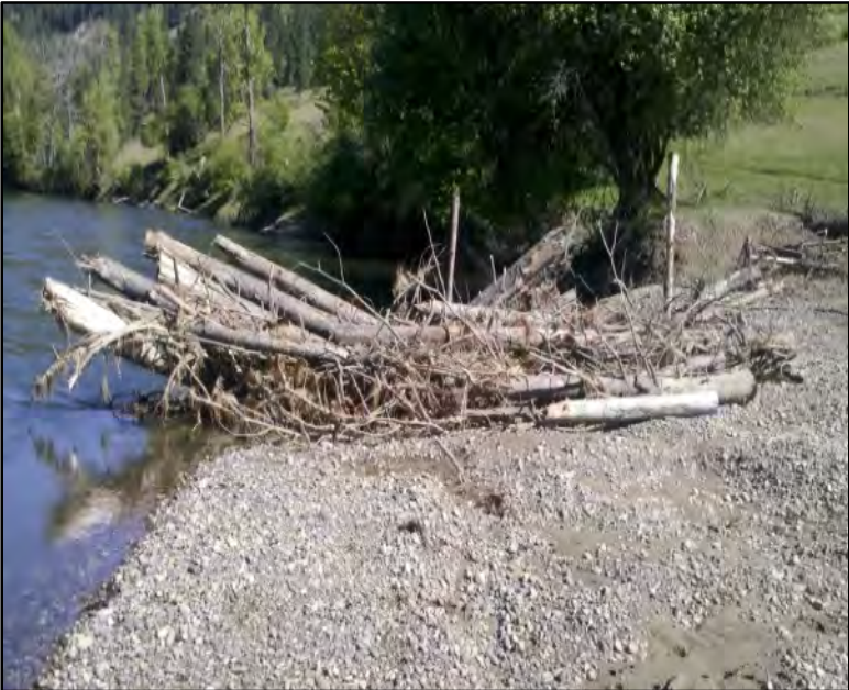
Figure 2-8. Examples of Type 2 Wood Bank Structures Immediately After Construction
