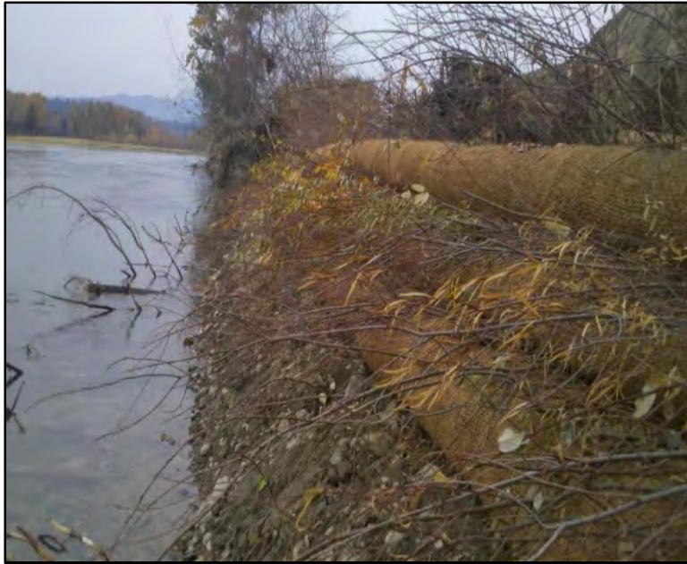
Recently completed soil lifts
