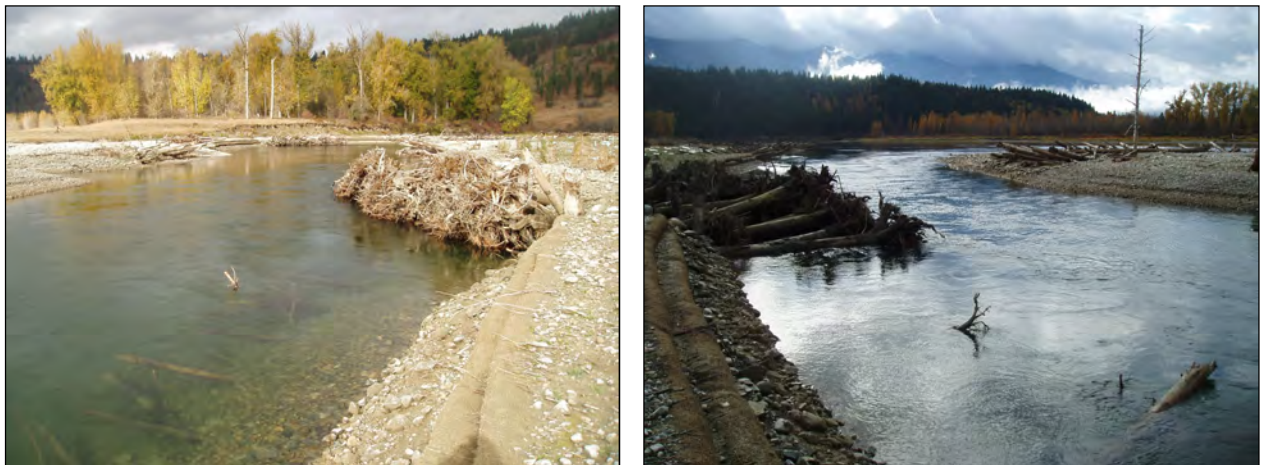
Figure 2-7. Type 1 wood structure immediately after construction.
