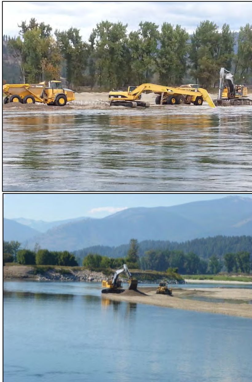
Figure 2-4. Examples of Pool Excavation
