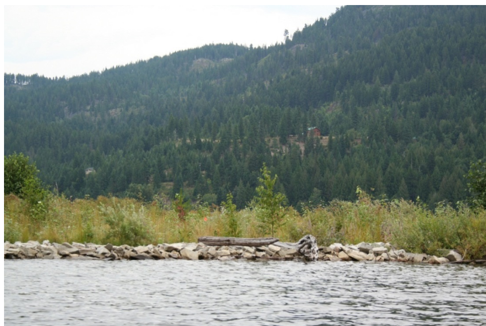
Figure C-8: Example of riprapped shoreline protection with woody debris and managed vegetation; Pack River nearly 5 years after establishment.
