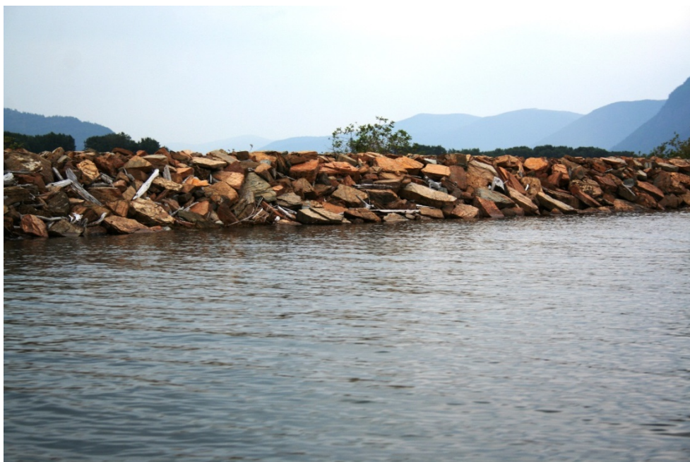
Figure C-7: Example of existing riprap breakwater at Area 3.
