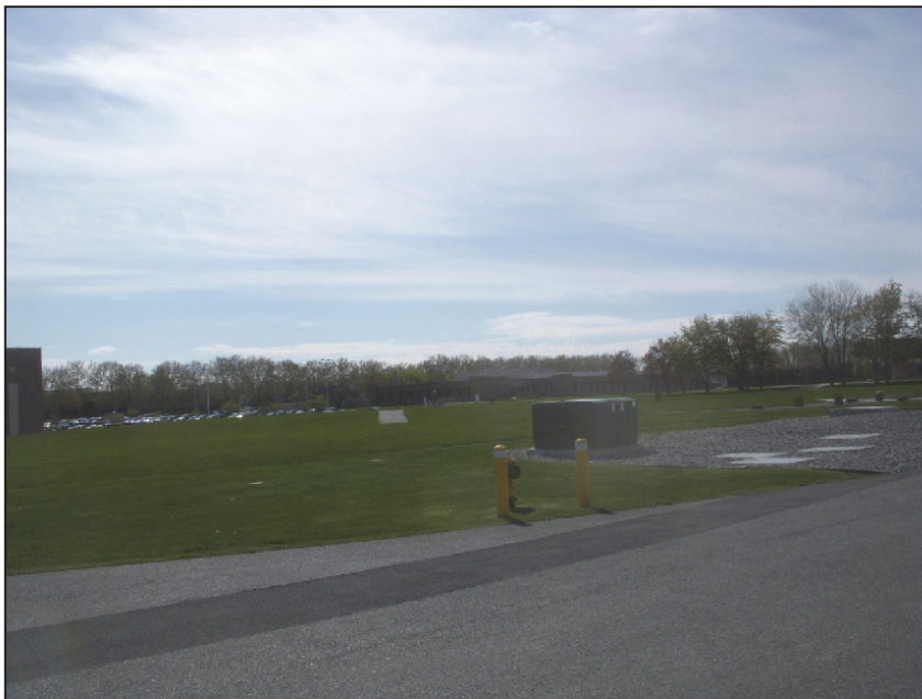
Photograph 4. APE between EMSL and BSF. Aspect: Southeast
