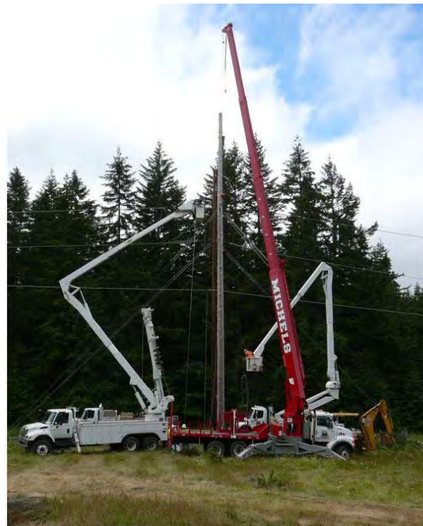
Figure 2-8. Installation of a Wood-Pole Structure
