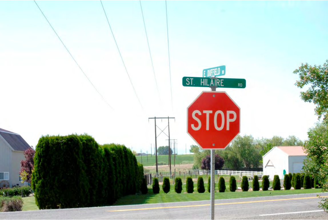
Figure 2-6. Existing Midway-Moxee Transmission Line in Area Without Adjacent Transmission Lines: Residential Area Near the City of Moxee
