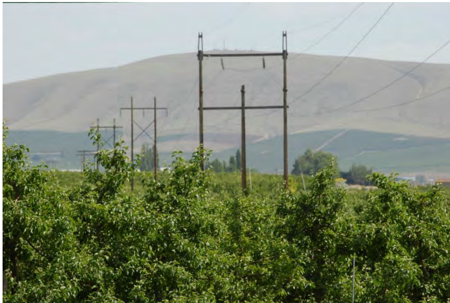
Figure 3.12-3. View of Midway-Moxee Line Mile 34 from Bittner Road
