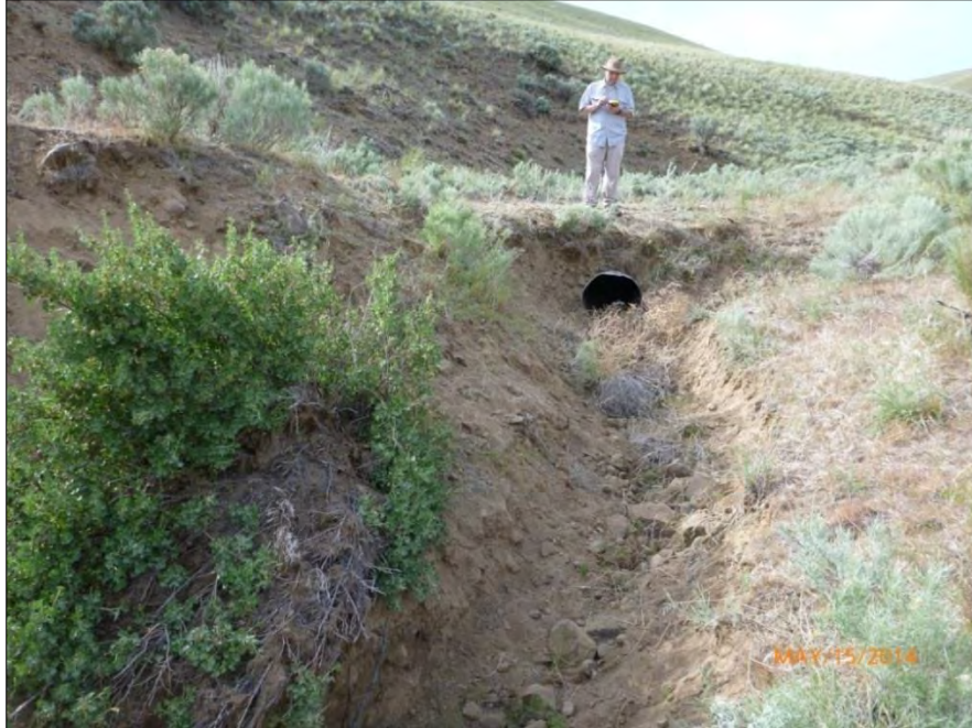
Figure 3.10-4. Photograph shows an existing culvert in an ephemeral stream between Midway-Grandview Structures 12/3 and 12/4 in Line Mile 12 that would be replaced. (Source: Tetra Tech 2014d)
