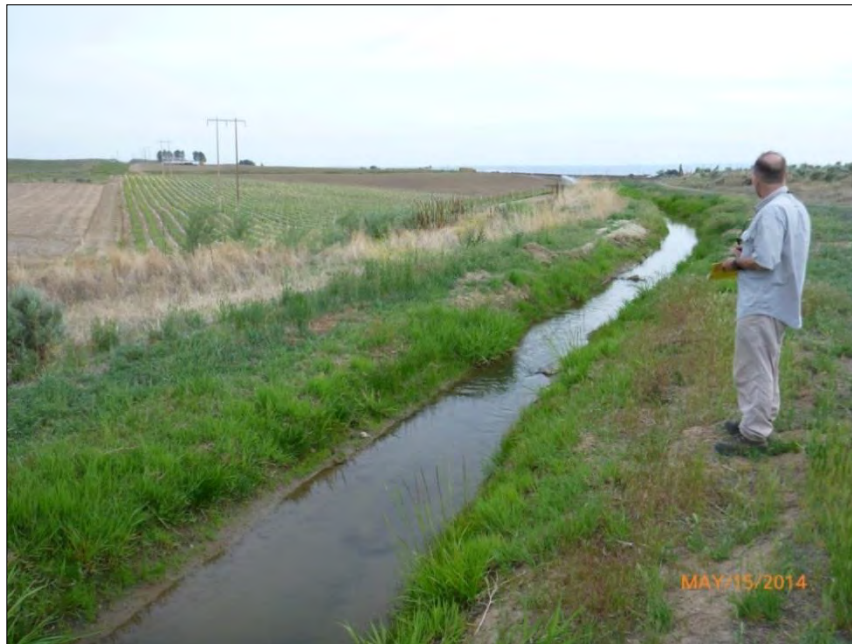
Figure 3.10-3. Photograph shows an irrigation ditch between Midway-Grandview Structures 23/5 and 23/6 in Line Mile 23 where a culvert would be installed for a new access road crossing. This ditch has been identified as a perennial waterway. (Source: Tetra Tech 2014d)
