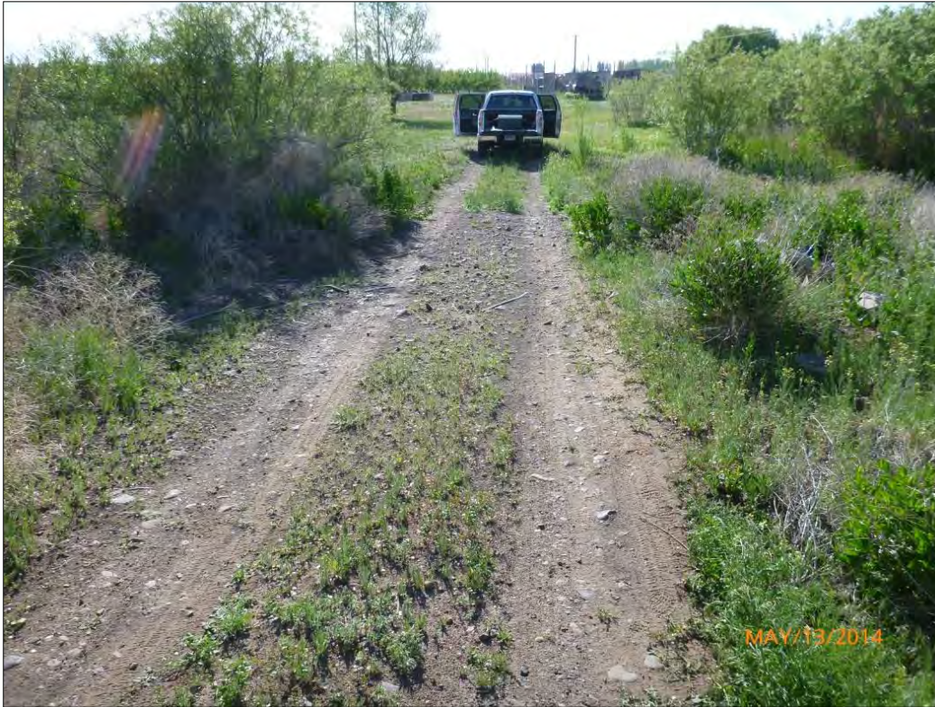
Figure 3.11-1. Photograph of Wetland Located Within Washout Gulch Between Midway-Moxee Structures 31/3 and 31/4 Showing Existing Agricultural Access Road that Crosses Wetland (Source: Tetra Tech 2014c)
