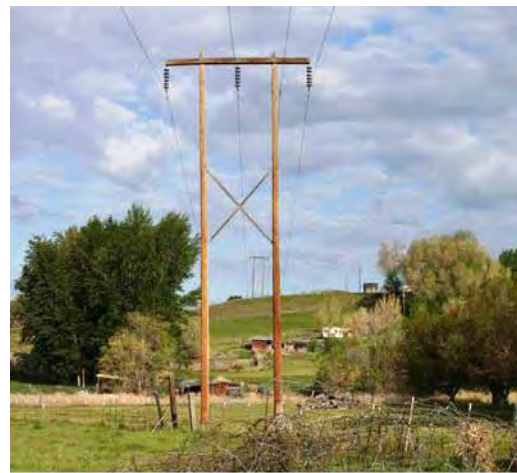
Figure 2-11. Danger Trees Near Midway-Moxee Structure 30/3
