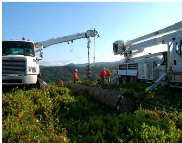
Figure 2-9. Augering a Hole for a Wood-Pole Structure
