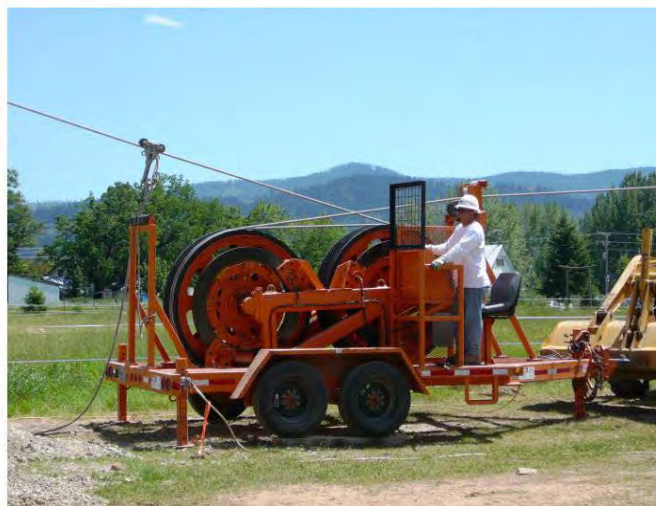
Figure 2-10. Tensioner Pulling Conductor
