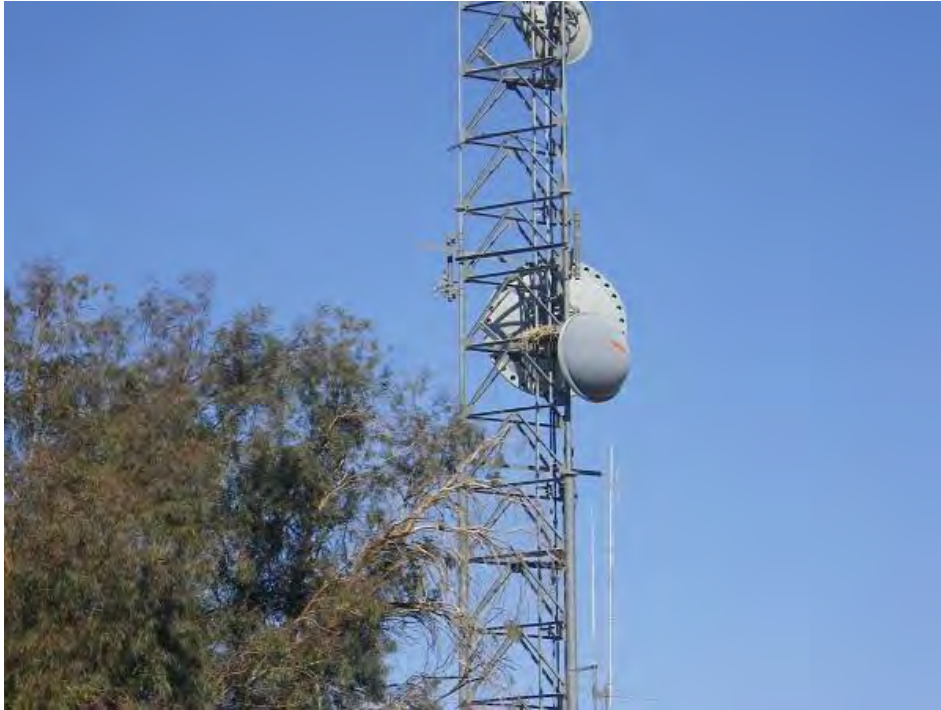
Photo 7: North-facing view of an active red-tailed hawk nest in a communication tower at the Gila Substation. Photo date: March 1, 2013.
