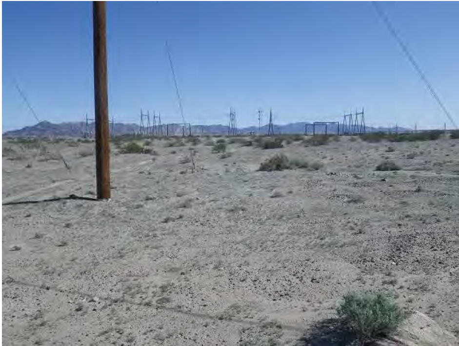
Photo 1: East-facing view towards the Gila North Substation from Gila-Knob 5-1, showing typical vegetation of the area. Photo taken on February 28, 2013.
