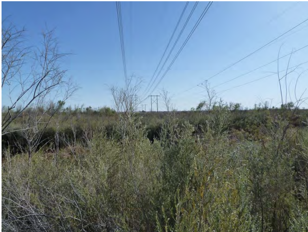
Photo 2 – View looking south at structures 2-6 and the span over the Gila River.
