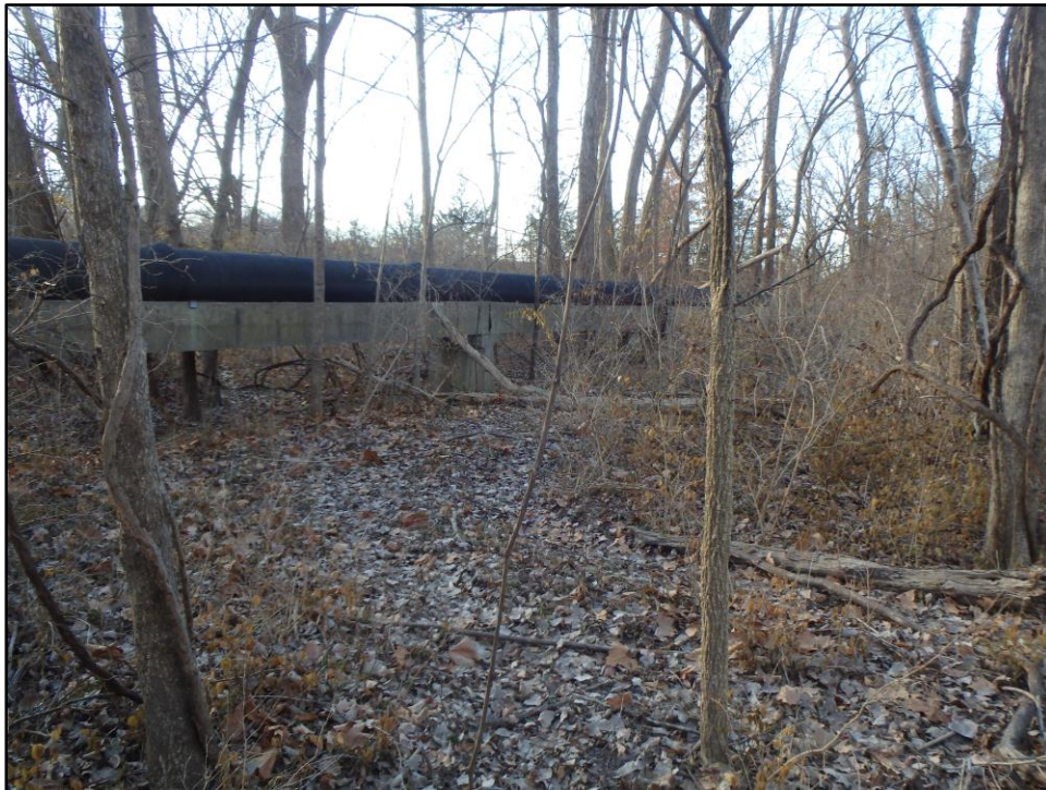
Photograph B-4: View of sewer line. Camera facing southeast.
