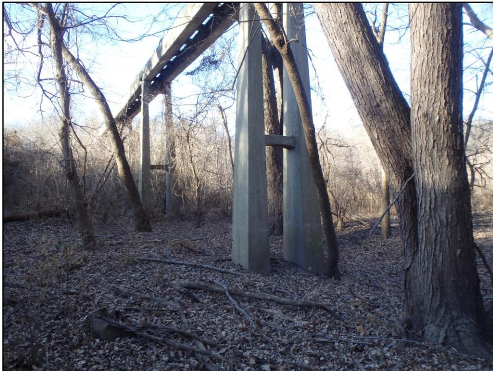
Photograph B-6: View of sewer line. Camera facing southwest.
