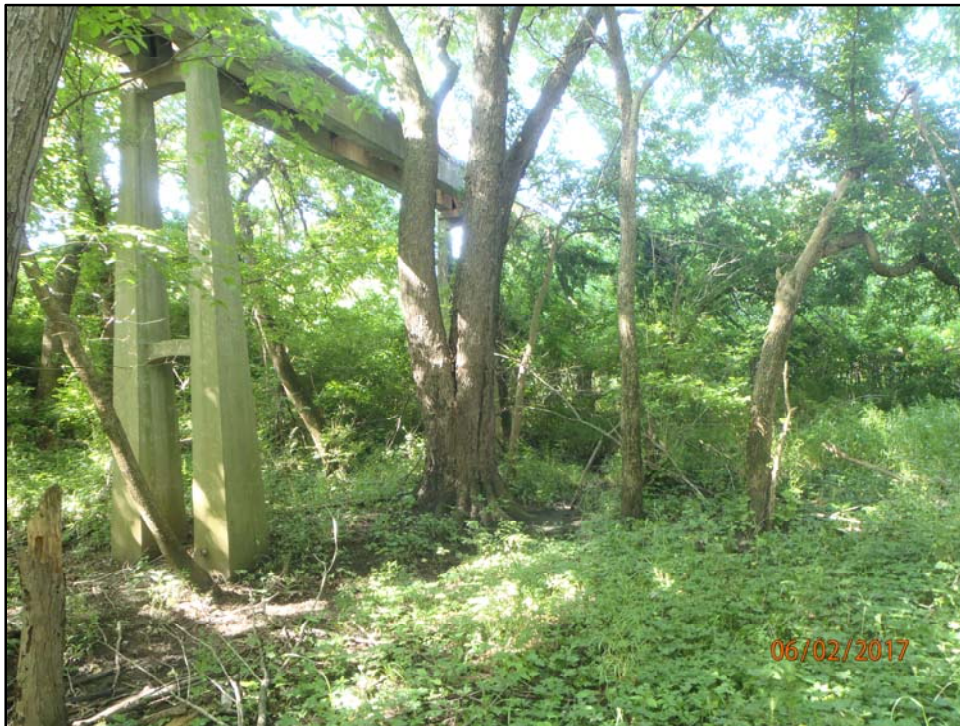
Photograph C-2: Trees near the sewer pipeline.
