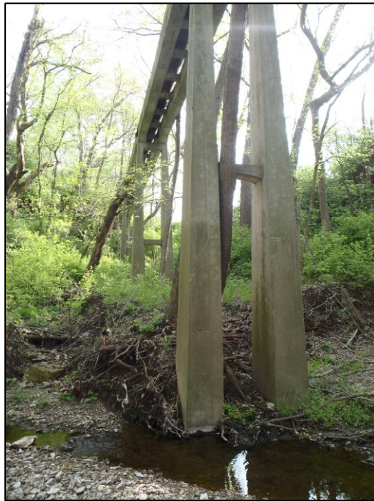
Photograph B-3: View of overhead sewer line. Camera facing northeast.
