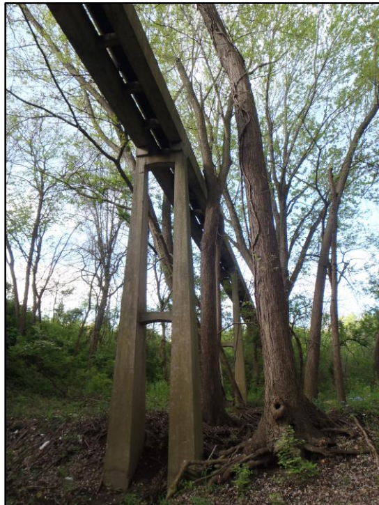
Photograph B-2: View of overhead sewer line. Camera facing southwest.
