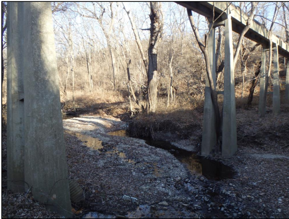
Photograph B-5: View of sewer line. Camera facing northwest.
