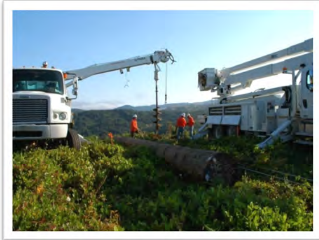
Figure 2-5. Auguring Holes for a Wood-Pole Structure
