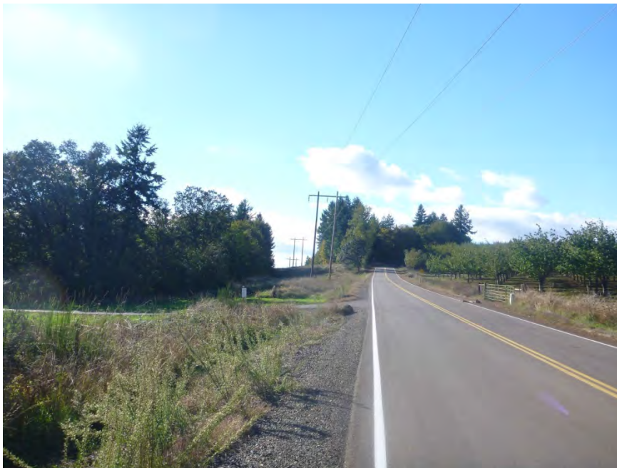
Figure 3-12. Salem-Albany No. 2, Facing Structure SA2:2/6 in a Residential Area of Salem
