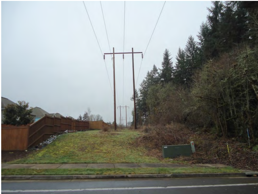
Figure 3-16. Viewpoint 1 - Existing View of Structure SA1:21/2, Looking South
