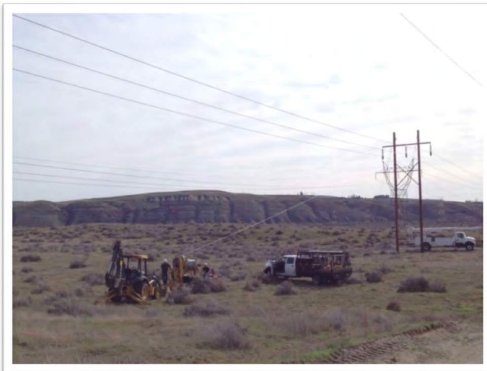
Figure 2-7. Conductor Tensioning after Conductor Installation
