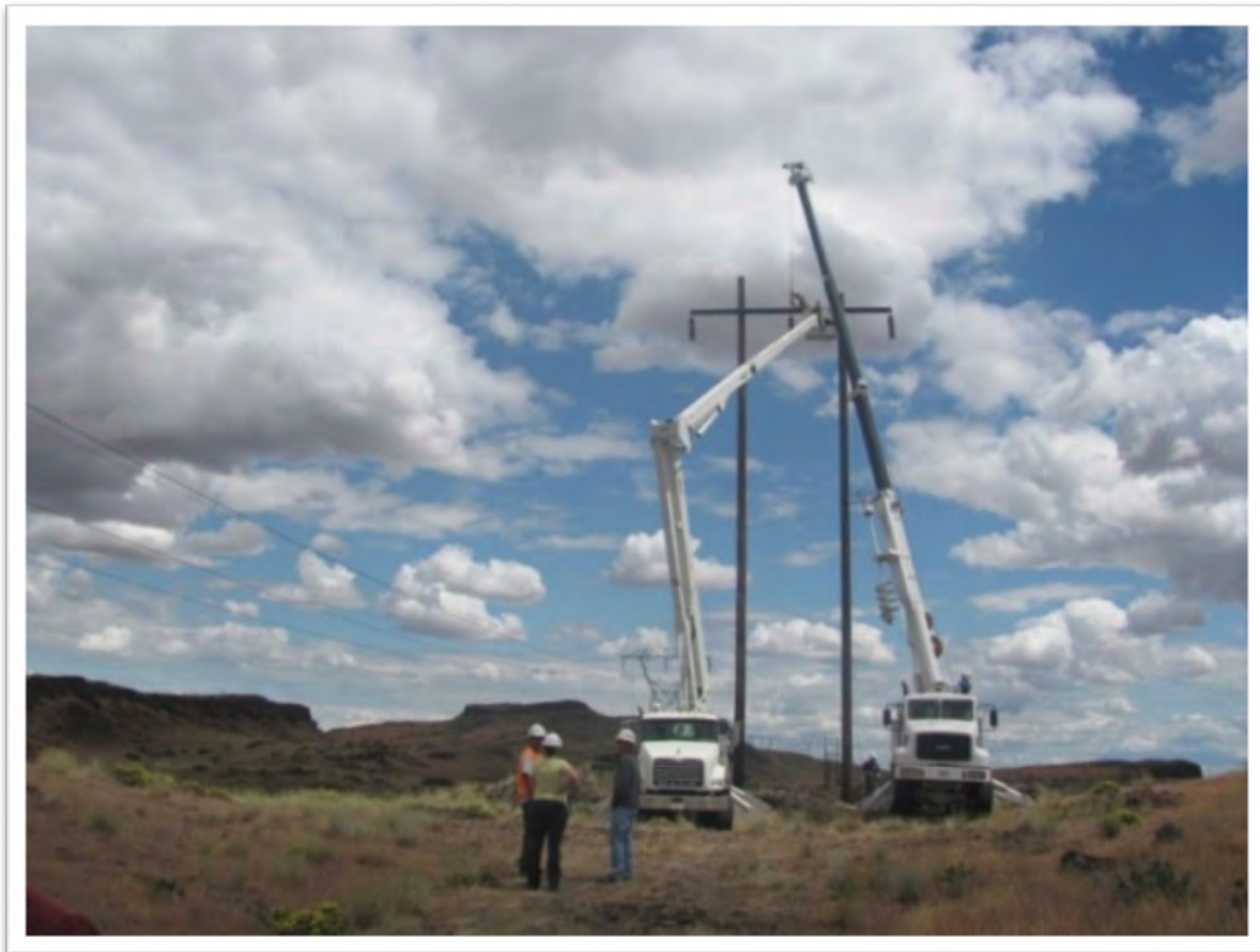
Figure 2-4. Removal of an Existing H-Frame Wood-Pole Structure
