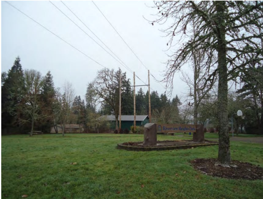
Figure 3-11. Structure SA1:12/5 in Riverview Heights Park, Looking North
