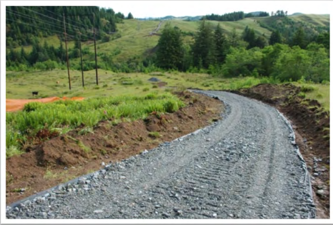
Figure 2-8. Improved Access Road
