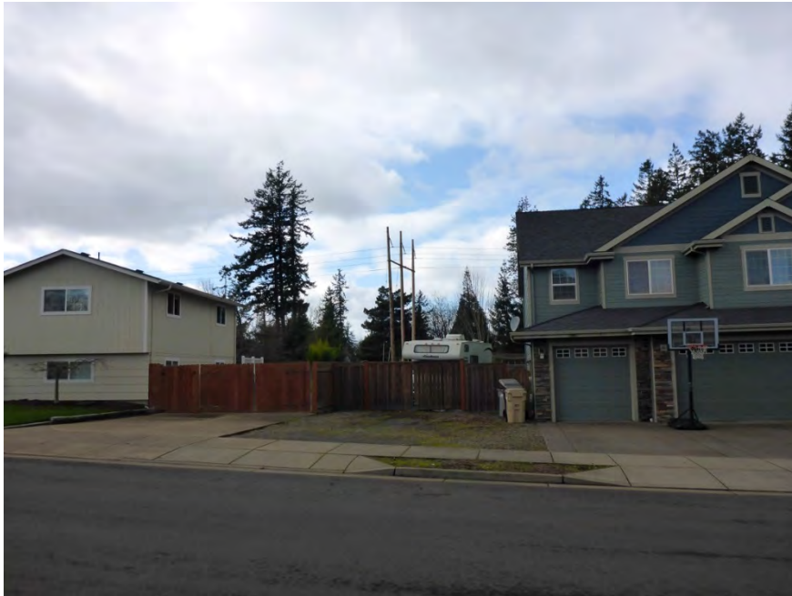
Figure 3-18. Viewpoint 2 - Existing View of Structure SA1:21/4, Looking West
