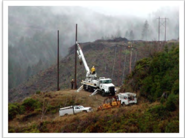
Figure 2-6. Installation of an H-Frame Wood-Pole Structure
