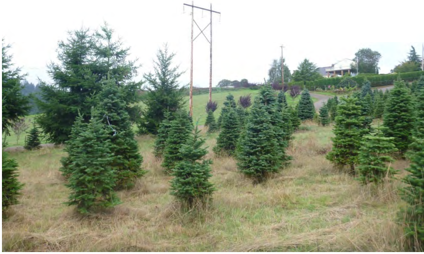
Figure 3-8. Transmission Line at Tree Farm, Looking at Structure SA1:6/8
