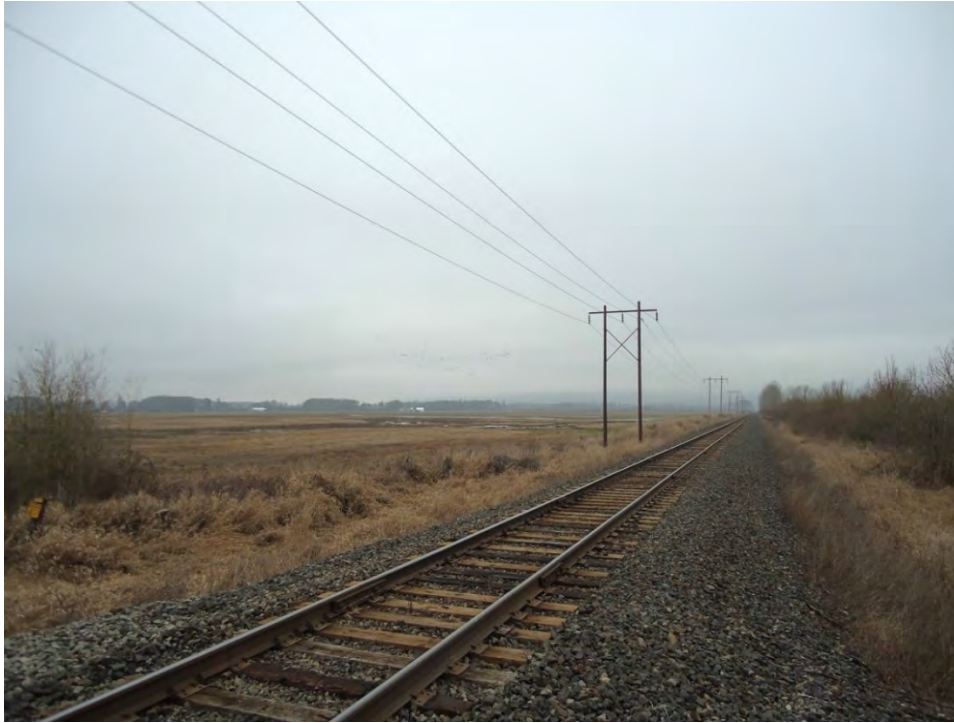
Figure 3a. View of Existing Two-Pole Wood Structures at SA1:12/3, Looking North
