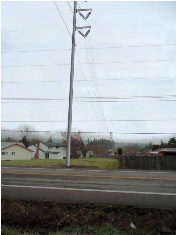
Figure 3-25. Viewpoint 5 - Proposed View of Structure SA1:21/8, Looking South
