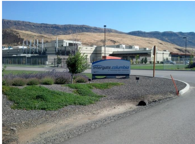
Photo 3.14-2. Intergate Columbia Technology Campus is one of the large technology centers in Douglas and Chelan Counties
