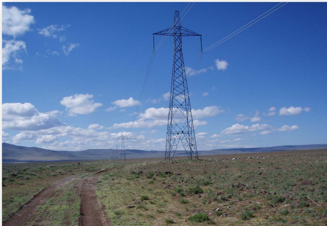
Figure 2.1-4: Existing PDCI Line BLM Land South of US 395 (Tower 220/2 looking south)
