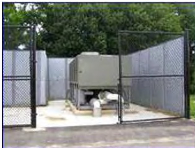
Figure C-4. HVAC outdoor concrete slab photo.
