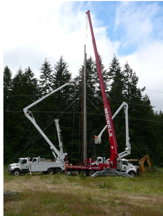
Photo 1: A wood structure being installed.
