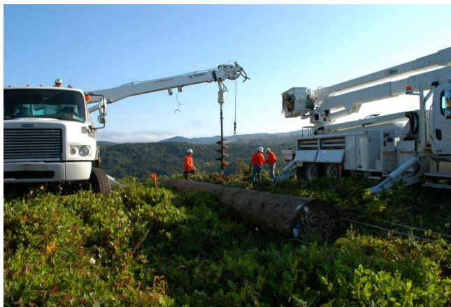
Photo 2: An auger in use attached to a drill rig.
