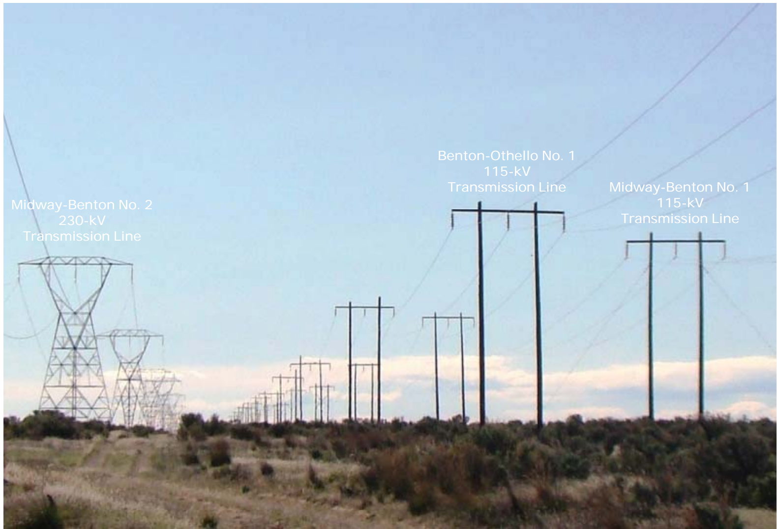
Figure 2-3. Existing Transmission Line Corridor
