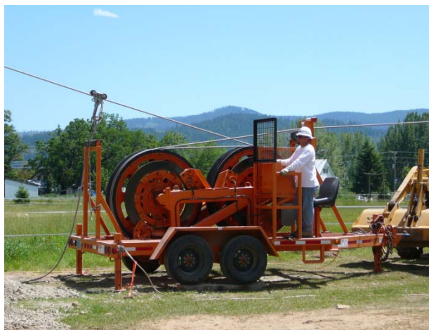
Photo 3: A tensioner pulling conductor.
