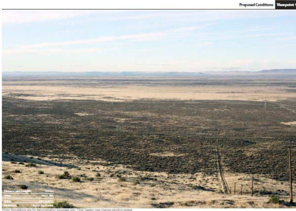
Figure 3.7-9. Existing (top) and Simulated View of the Midway Benton No. 1 and Midway Benton No. 2 Transmission Lines from East Gable Mountain under the Proposed Action. Due to distance and dark background, the wood structures are minor visual elements within the landscape.
